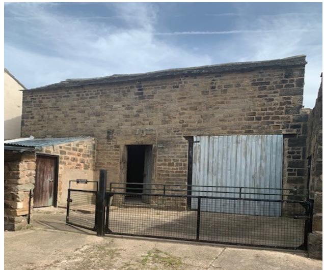
Fig 3 – Barn: Rear – as viewed from courtyard side looking north.
