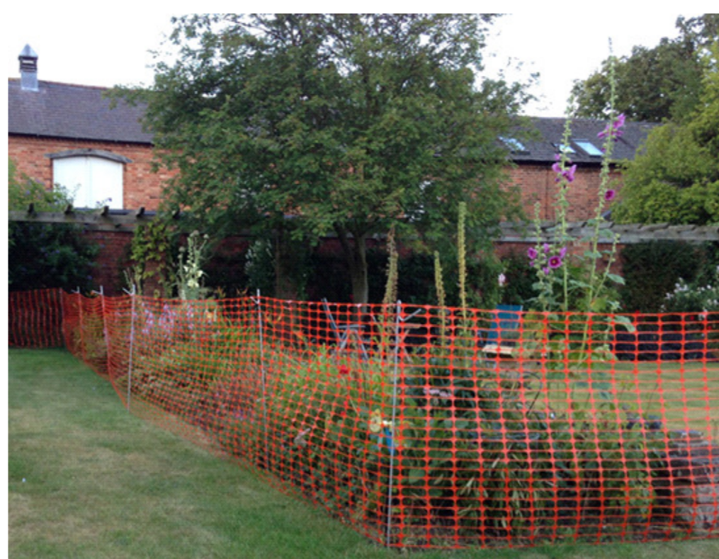
Plastic mesh tree protection fencing
