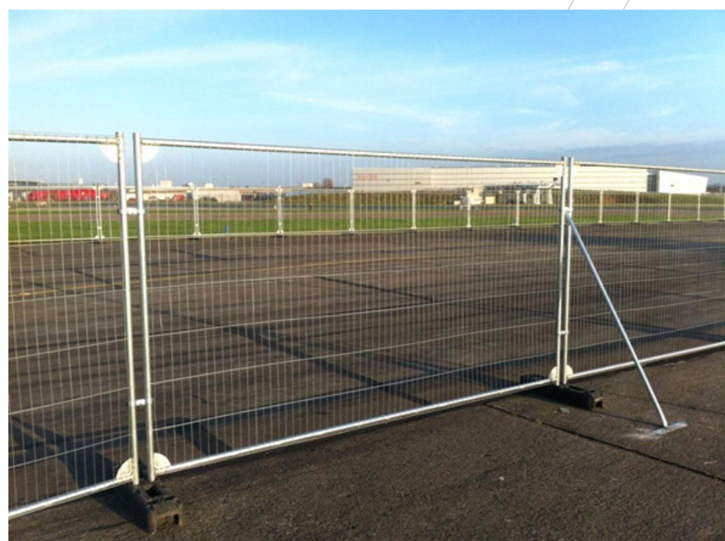
Heras tree protection fencing
