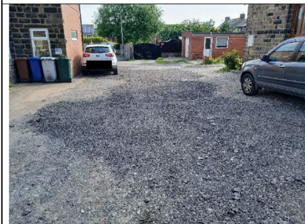
Photo 11: Developed land access road.
