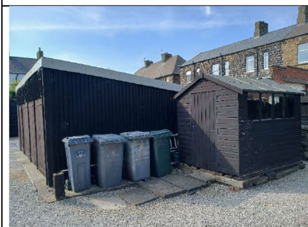
Photo 9: Buildings and developed land on site.
