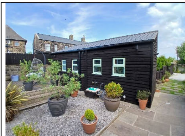
Photo 7: Buildings and developed land on site.
