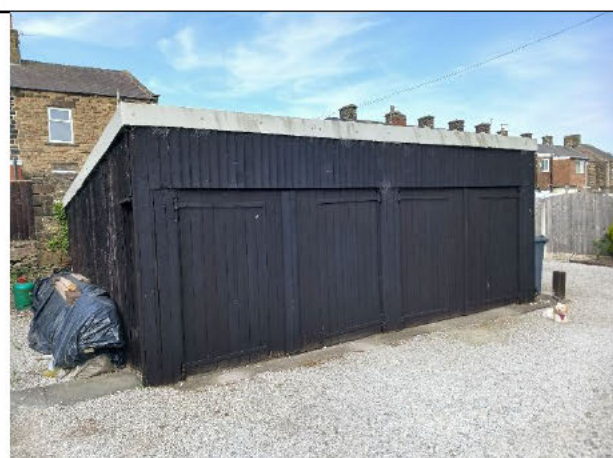
Photo 10: Buildings and developed land on site.
