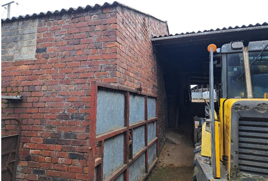
Plate 1: Image showing B3 (left) and sheltered walkway between B3 and B4
