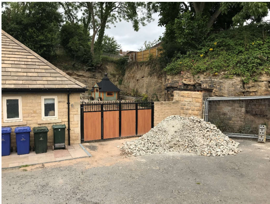
Fig 04. View of site from site access looking north towards parking area beyond gates.
