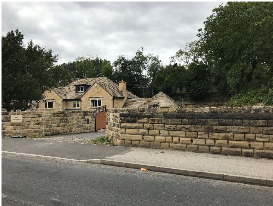
Fig 02. View of the site frontage and extg dwelling looking NWest from Common Road.
