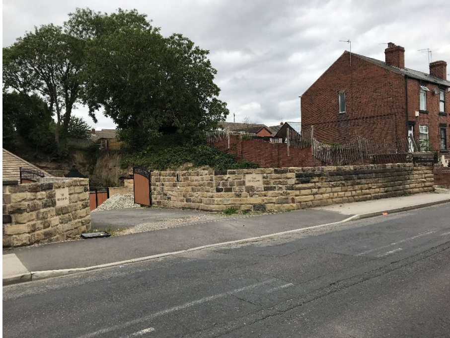
Fig 01. View of the site and access from Common Road looking North
