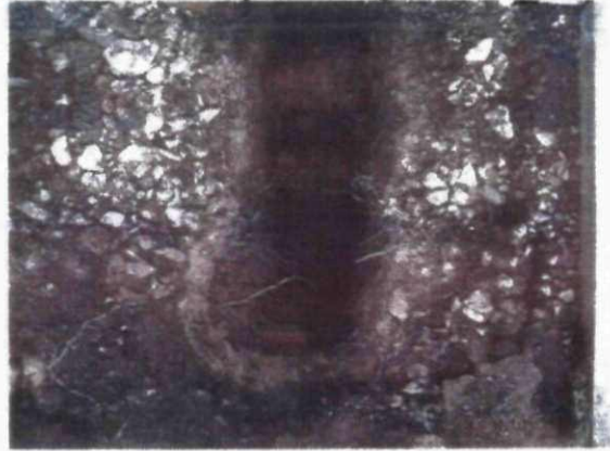
Photo 2 – Close up of footing in TP/BH1a.
