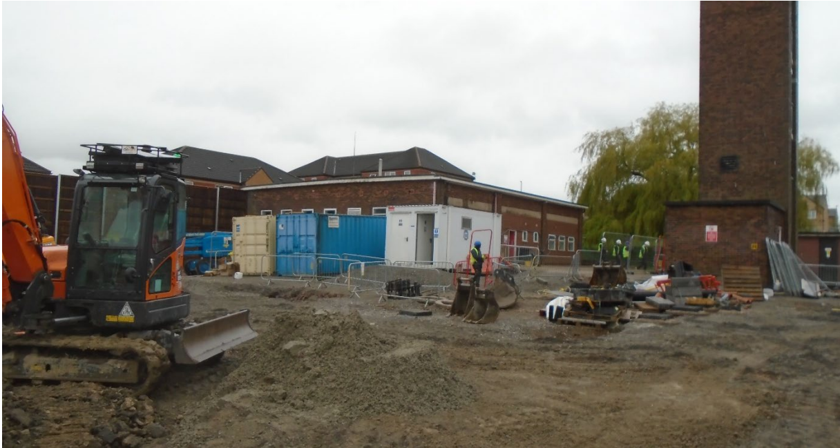
5. View across drill yard – (note, acoustic wall to left)
