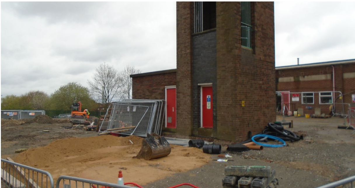
4. View to wards Drill yard (Drill yard to the left of tower building)
