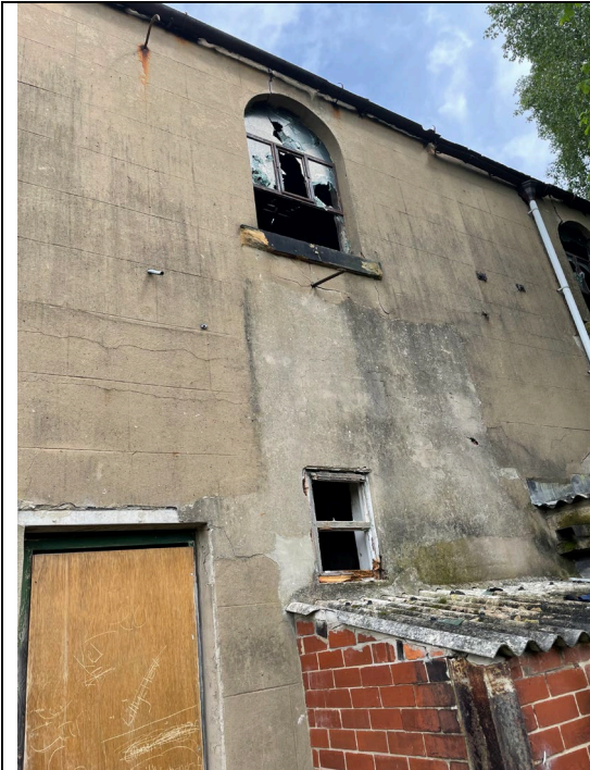
9. Main Building Rear Elevation
