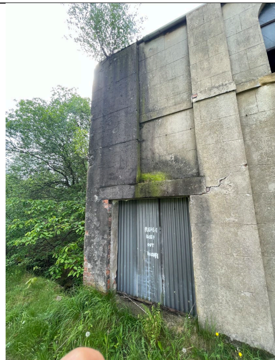
4. Main Building Front
