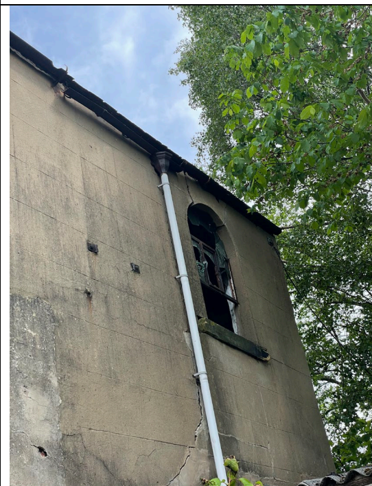
8. Main Building Rear Elevation
