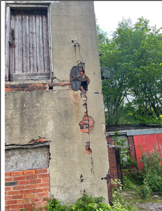
5. Main Building Right Elevation
