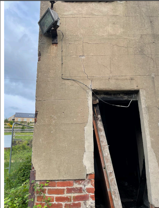
6. Main Building Rear Elevation
