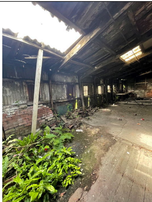
15. Inside Rear Bays
