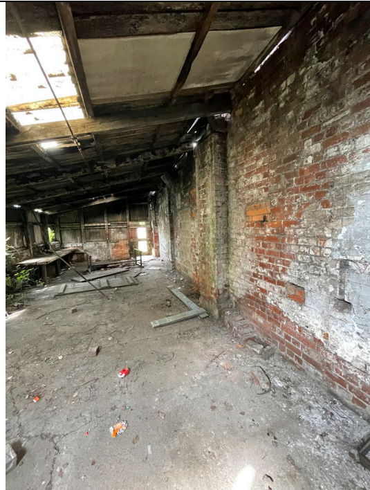
17. Inside Rear Bays
