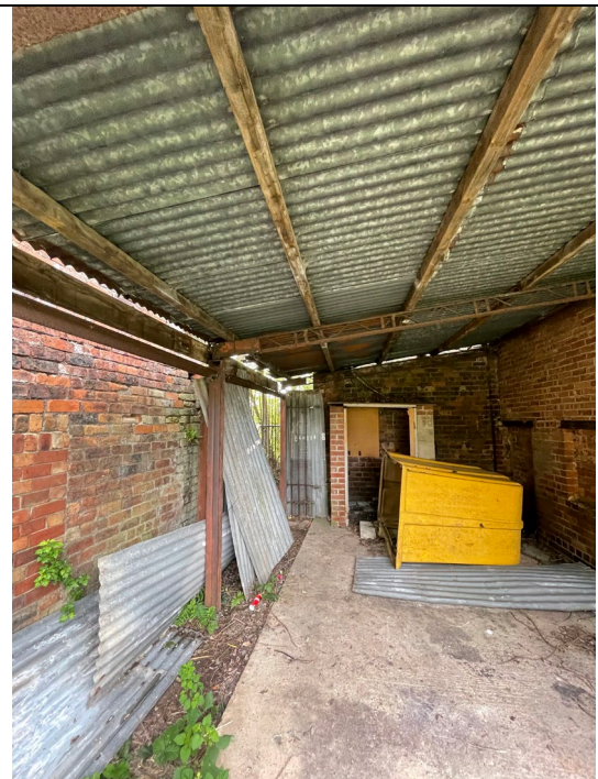
12. Inside Rear Bays
