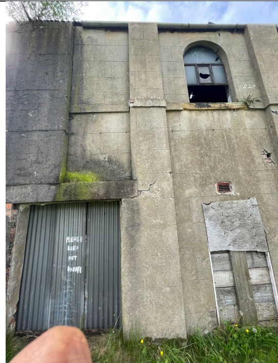
2. Main Building Front
