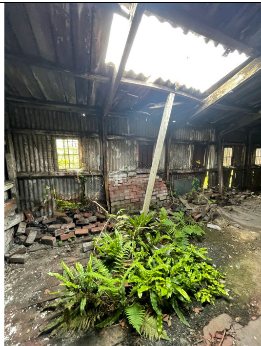
16. Inside Rear Bays
