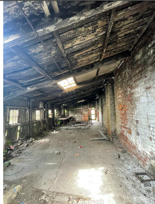
18. Inside Rear Bays
