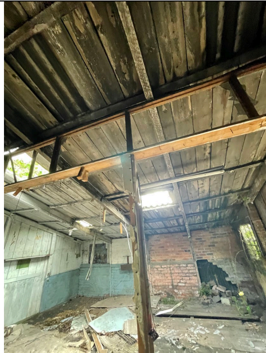
13. Inside Rear Bays
