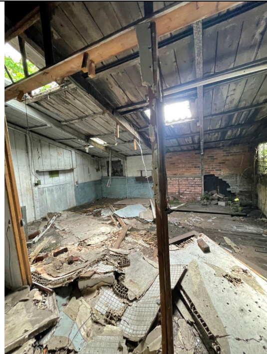
14. Inside Rear Bays
