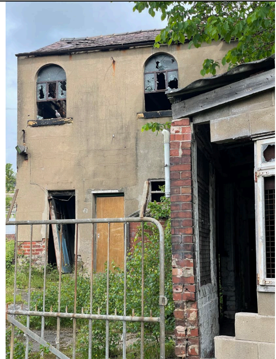
10. Main Building Rear Elevation
