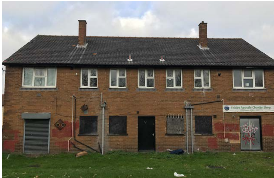
View of Rear Elevation
