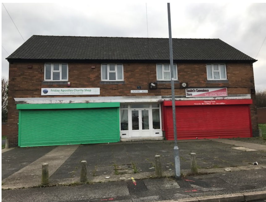
View of Existing frontage
