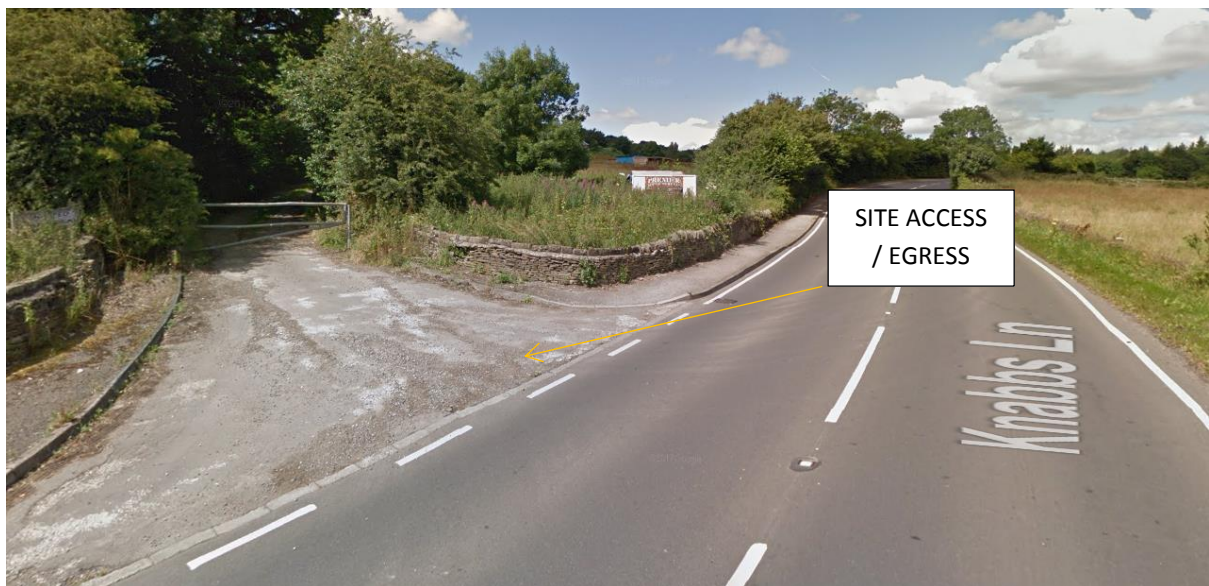
Photo 1 – Looking North along Knabbs Lane (B6449)
