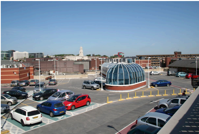
The roof level with rooflight
