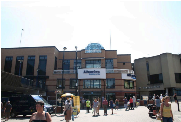
Cheapside Entrance to The Alhambra Shopping Centre
