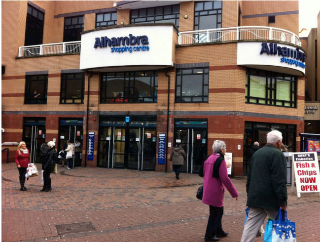
Cheapside Entrance : A weak entry point to the Centre
