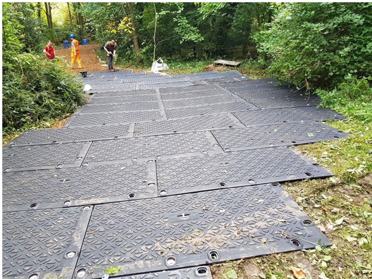
Figure 6: Ground protection boards
