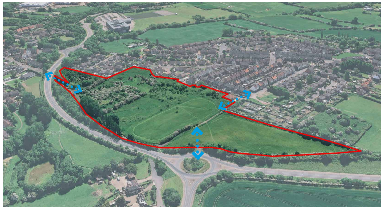
Site Aerial showing site access points.
