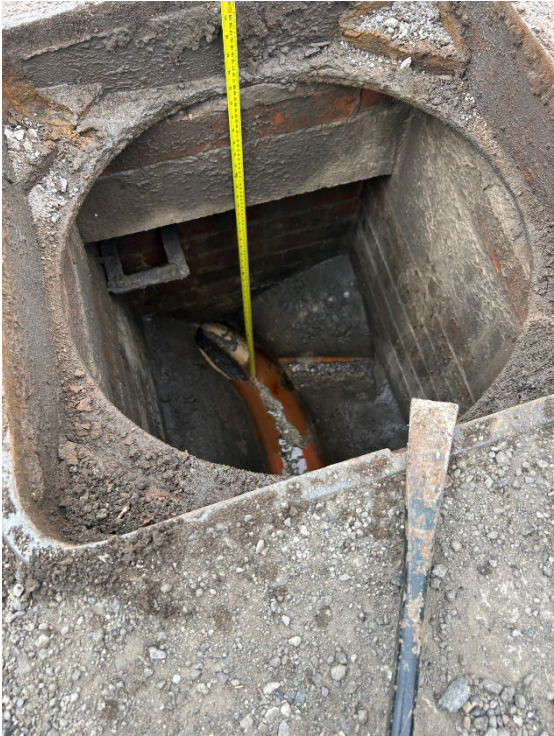
Figure H1 – Combined Sewer Manhole (Open)
