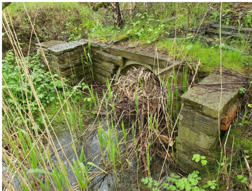
Outfall Headwall during RWD site visit May 2021 (prior to debris removal)
