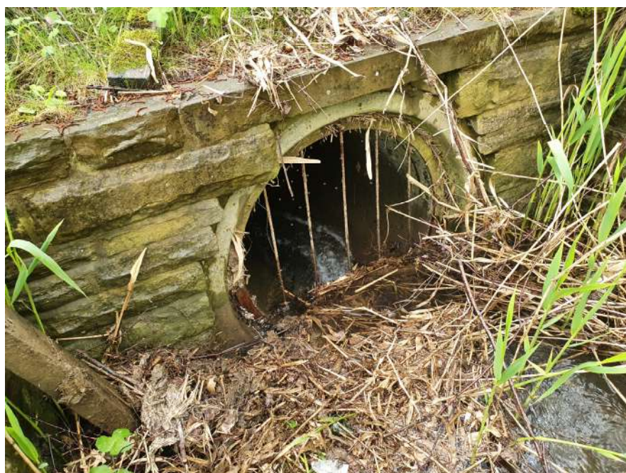
Outfall Headwall during RWD site visit May 2021 (following debris removal)
