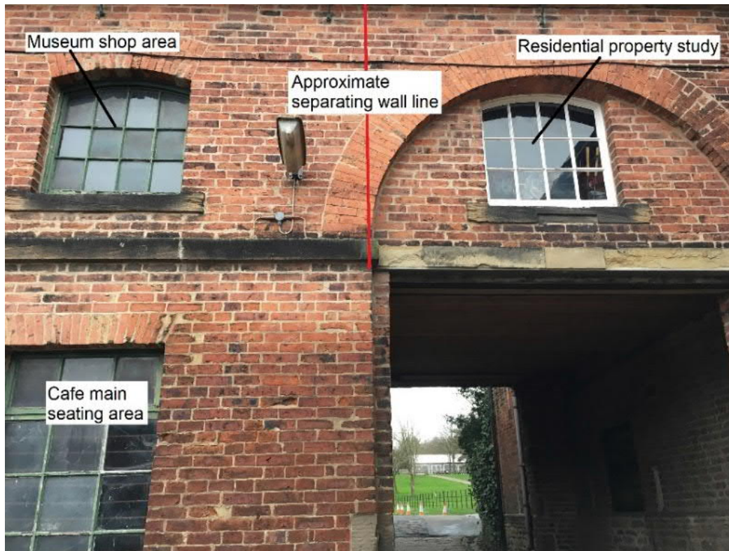
Figure 1: Courtyard elevation of stable block building and adjoining residential property
