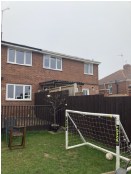
7 View to 12 Carlton Street
