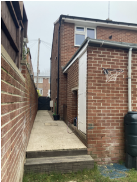
2 Side passage and outhouse
