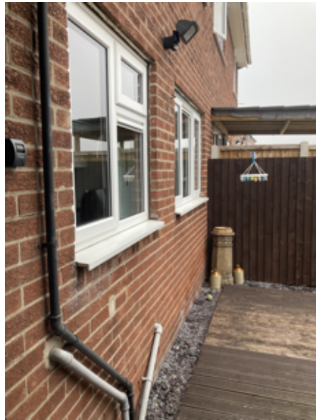
4 Rear windows and decking
