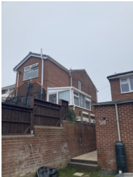
6 View to 8 Carlton Street
