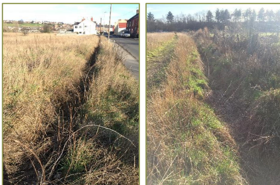
Right: Drain 1. Left: Drain 2.
