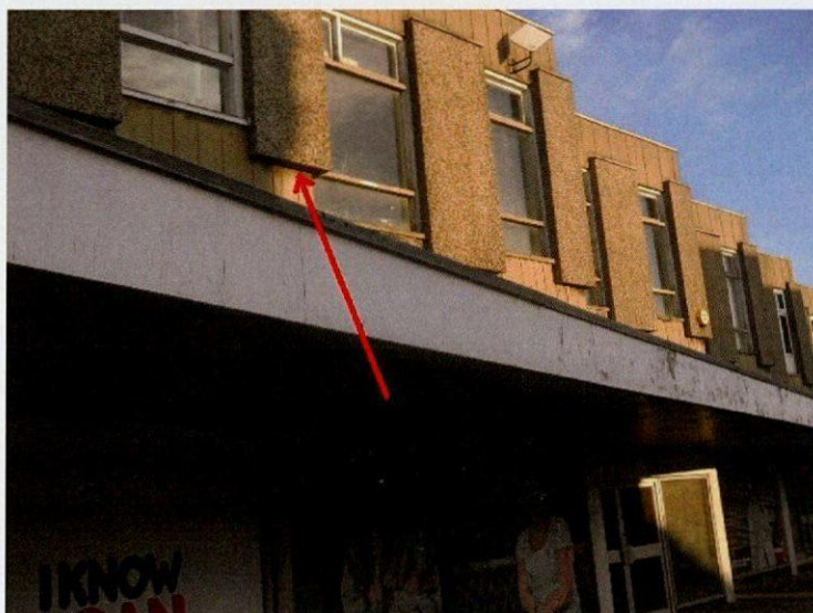
Plate 1 – Indicating potential roosting locations behind concrete cladding
