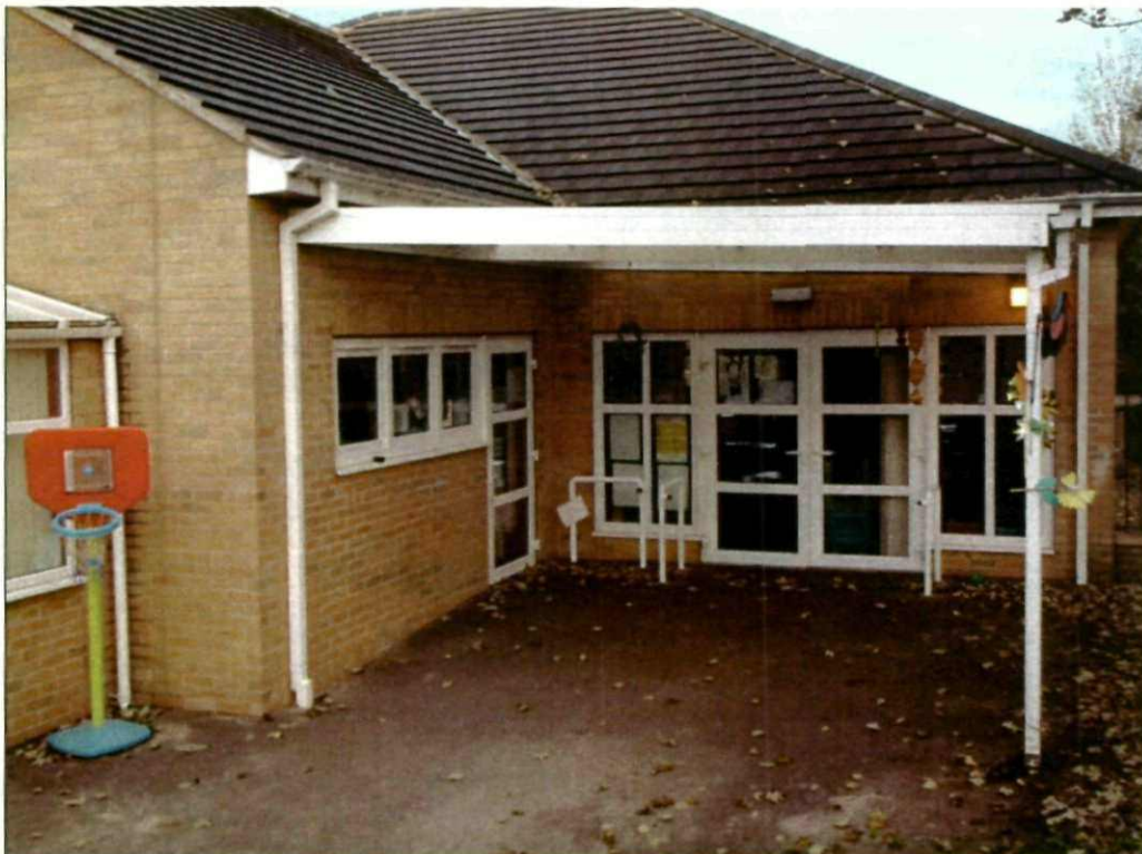
Photo No. 3 – Elevation showing existing canopy and side of lean to where new canopy is proposed.
