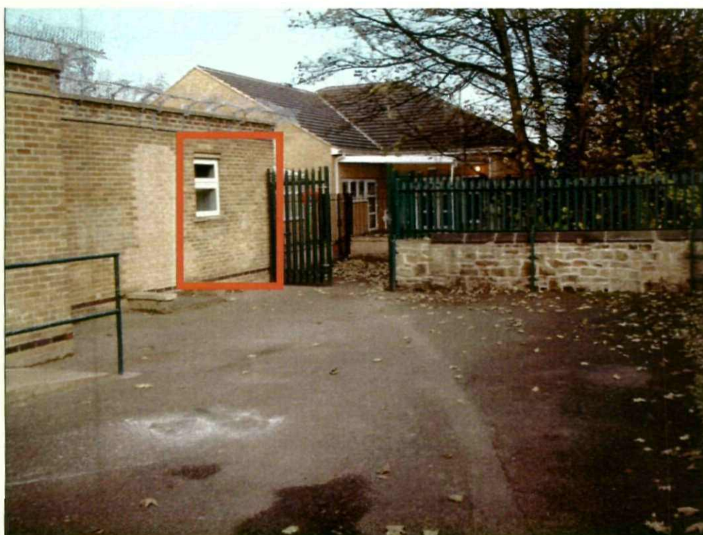
Photo No. 4 – Elevation showing location of new proposed door way and access into school.
