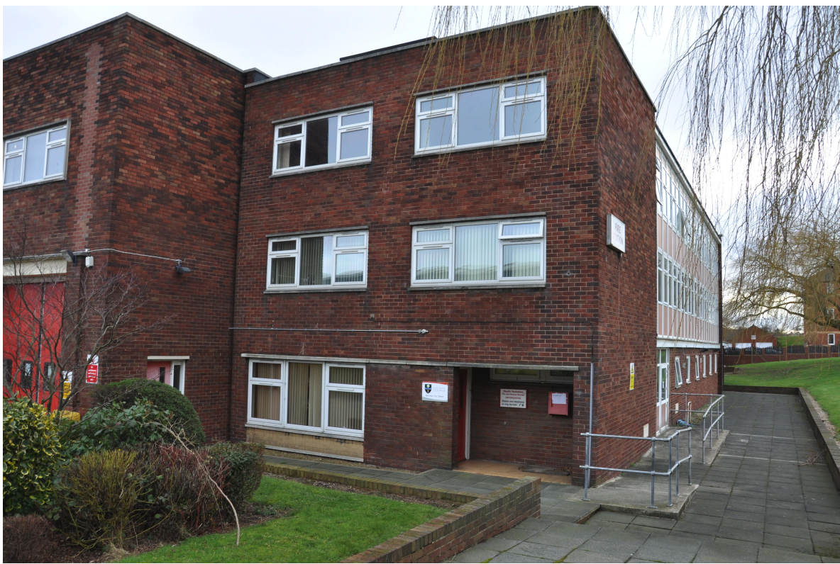
VIEW 01 - Existing Fire Station to be demolished.
