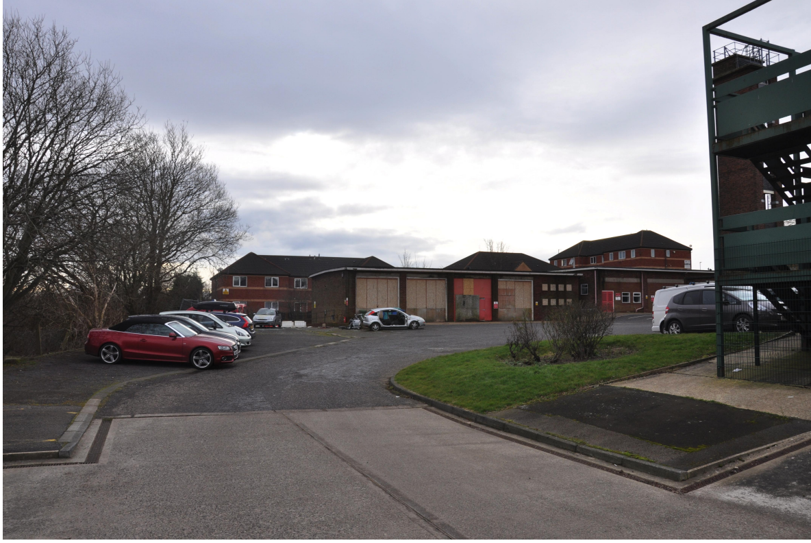
VIEW 04 - Existing Garage Building to be demolished.
