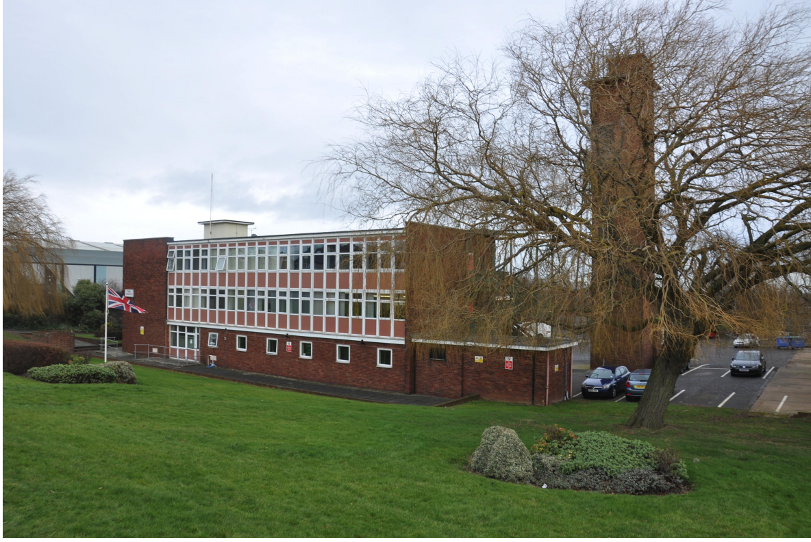
VIEW 05 - Existing Fire Station to be demolished.
