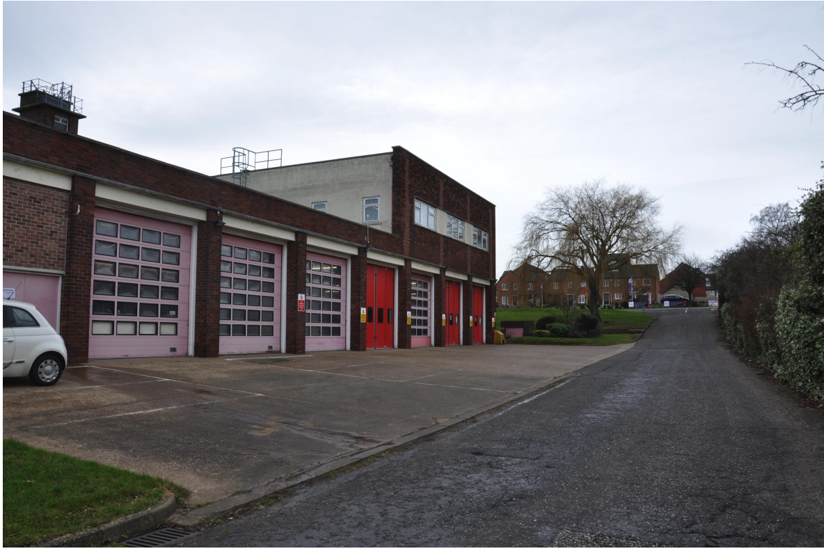
VIEW 03 - Existing Fire Station to be demolished.
