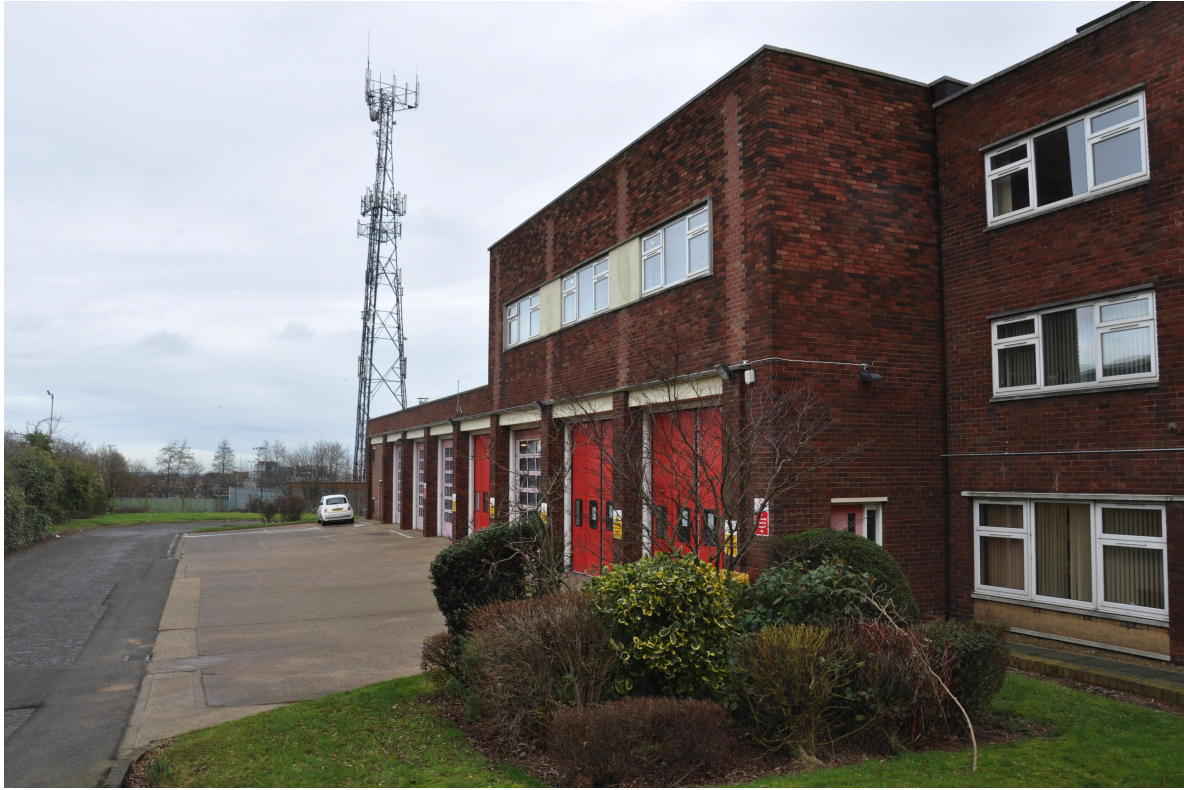
VIEW 02 - Existing Fire Station to be demolished.
