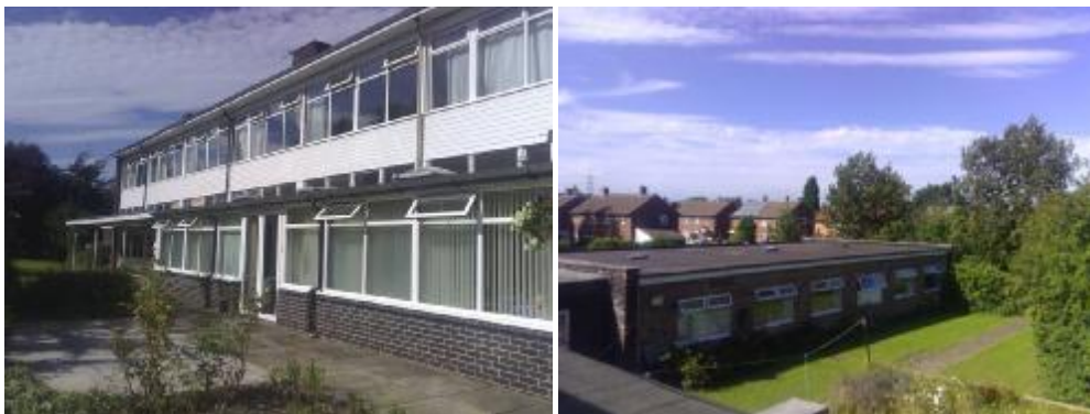
Central two-storey building (Left), single-storey wing (Right)
