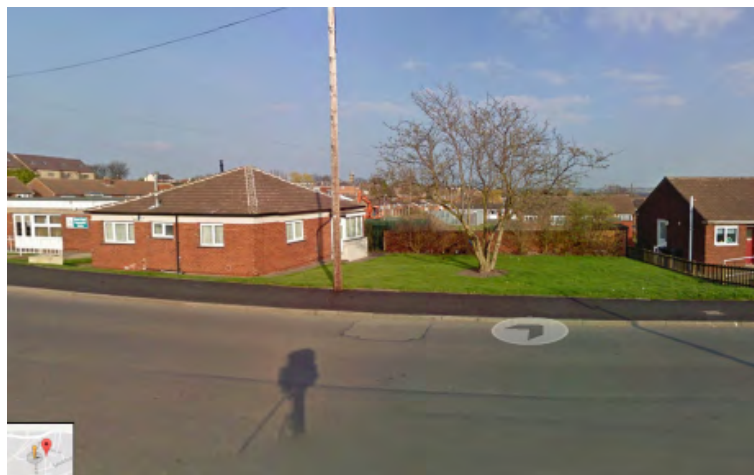
2 View of site from Manor Grove
