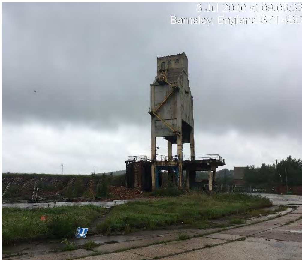
Photo 2: Remaining tower associated with the coking ovens.
