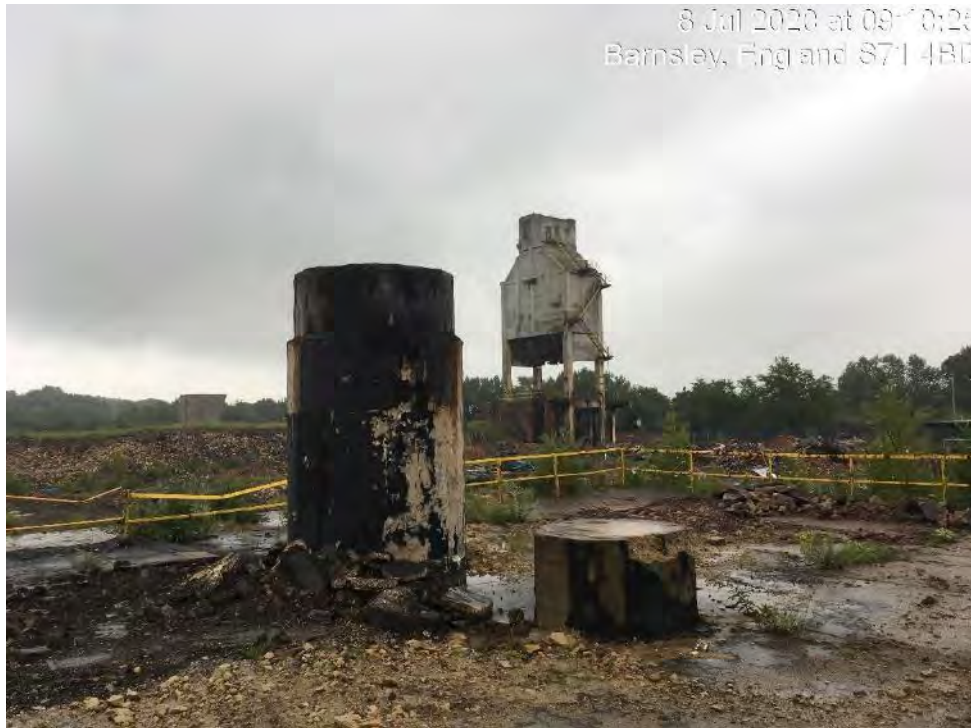
Photo 3: Small stack in the production area with coal tar staining.
