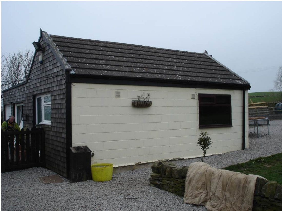
04. View of south east elevation of outbuilding.
