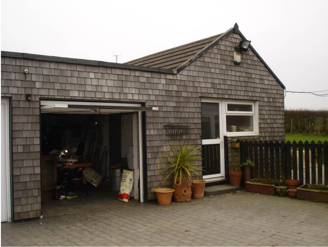
03. Part view of south west elevation of existing outbuilding.
