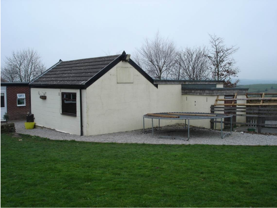
05. View of north east elevation of outbuilding.
