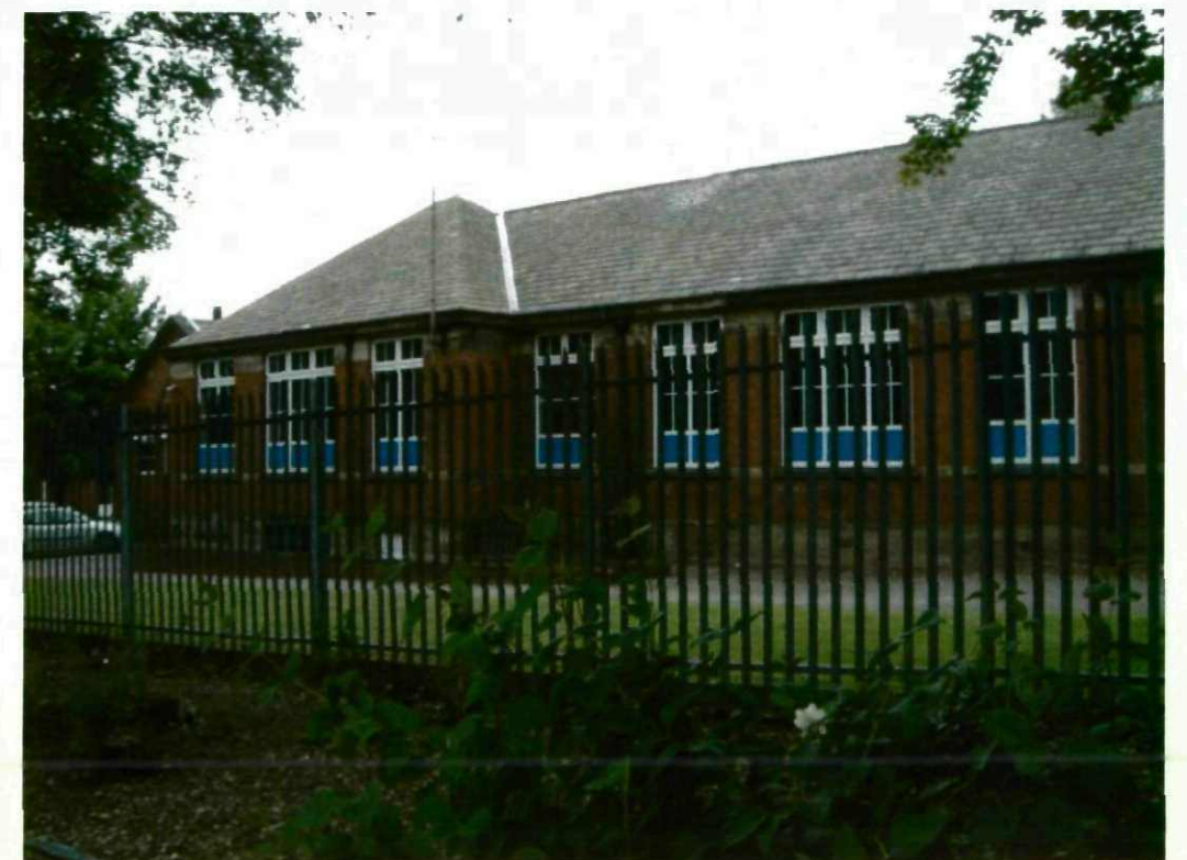
Existing School buildings to Kirk Balk Street
