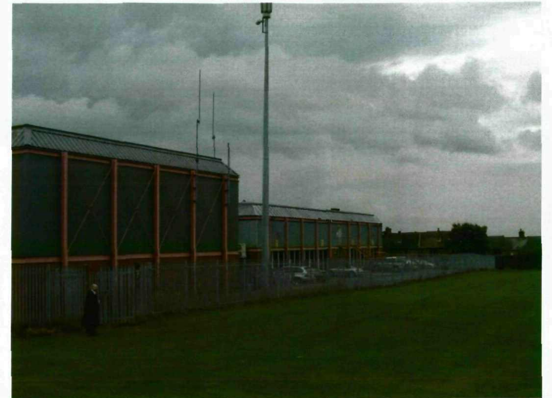
External View of Hoyland Leisure Centre and playing fields to West of Site
