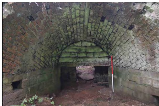
Figure 19: East tuyere arch (1m scale)
