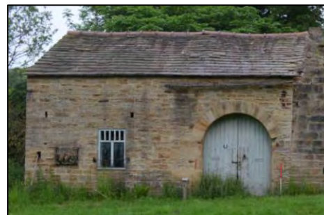
Figure 24: South-west elevation of Casting Shop
