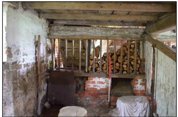
Figure 30: Detail of south-east cowstall (1m scale)
