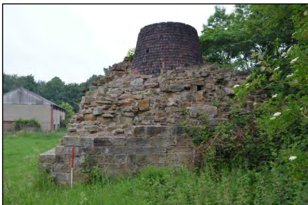
Figure 17: South elevation of furnace (1m scale)
