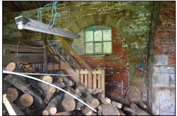
Figure 28: Blocked arched door in east of haymow
