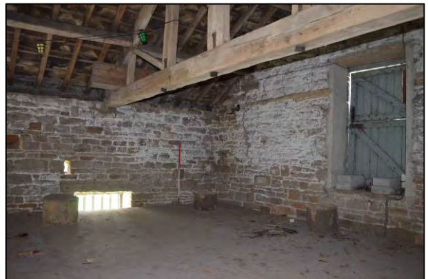
Figure 32: View of the loft (1m scale)
