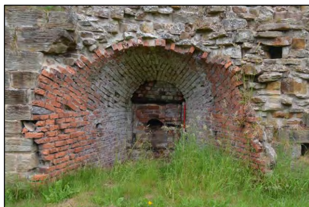
Figure 20: Secondary west tuyere arch
