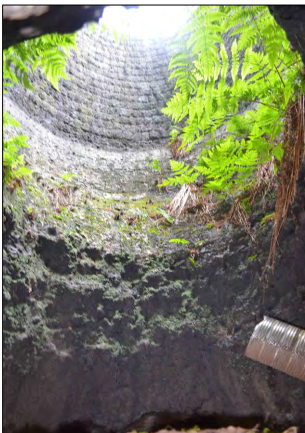
Figure 22: Interior of furnace, looking south-west
