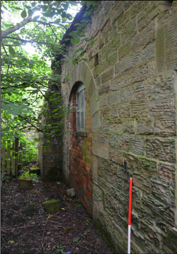
Figure 26: North-east elevation of Casting Shop
