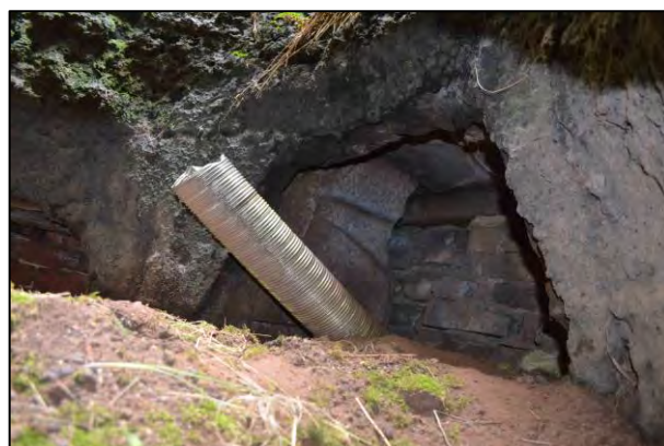
Figure 23: Interior of rear blocking to work arch
