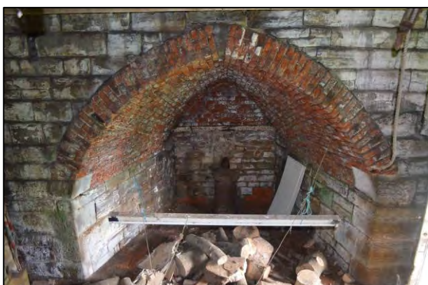
Figure 18: North work arch in adjoining building
