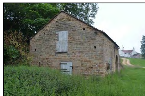
Figure 25: North-west elevation of Casting Shop
