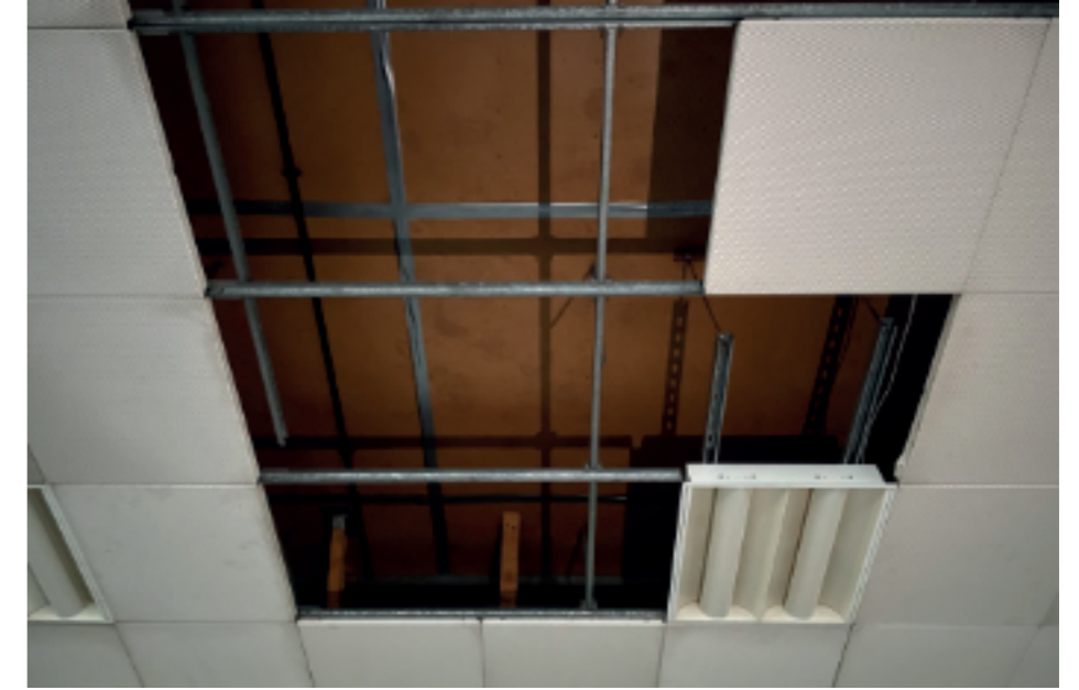
Computer Hall inserted ceiling structure revealed
