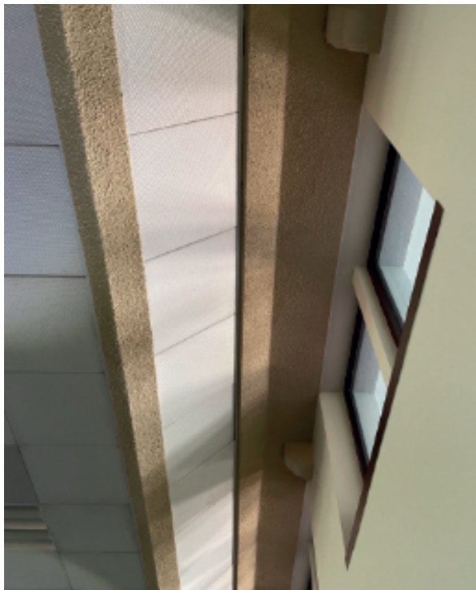
Computer Hall suspended ceiling junction
