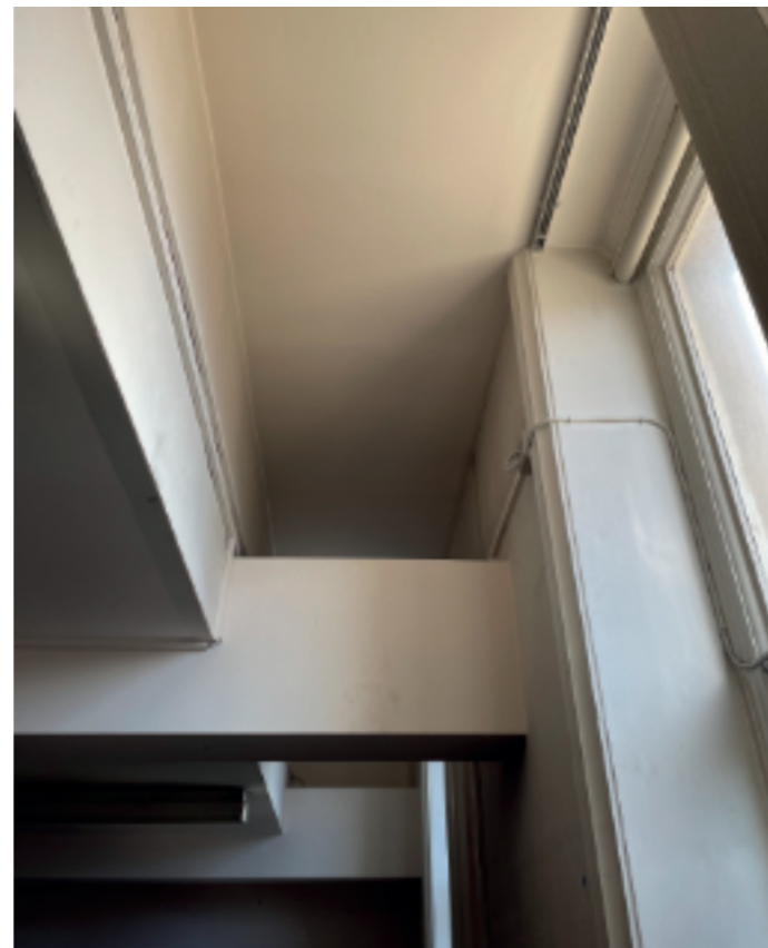
Inserted mezzanine floor supporting structure
