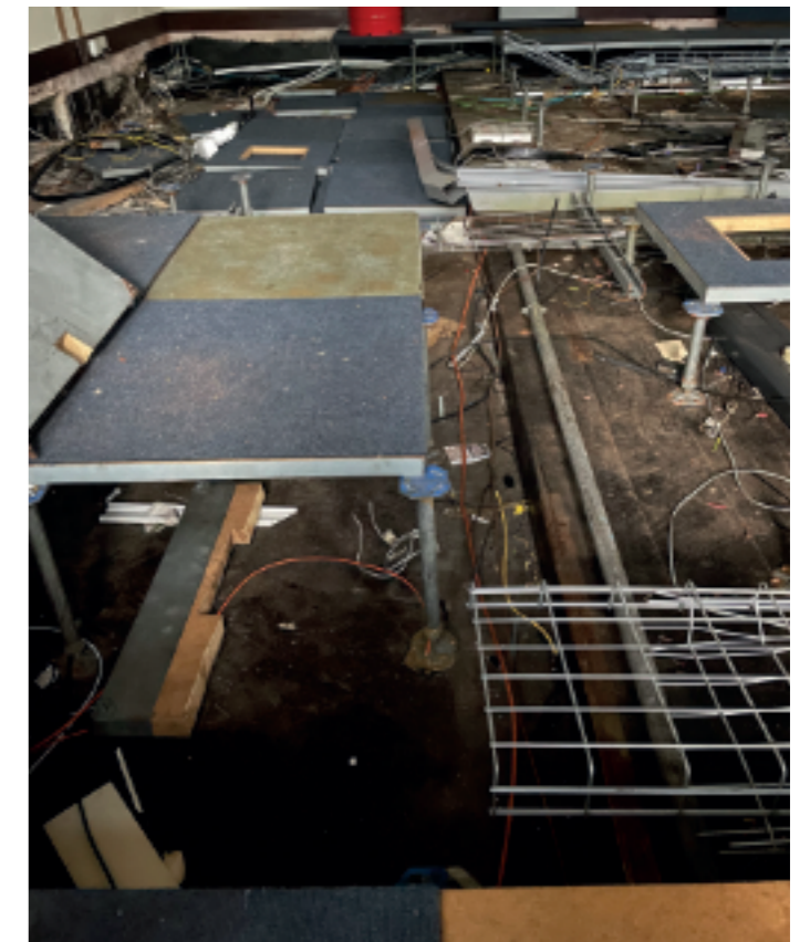
Court Room floor finishes visible?
