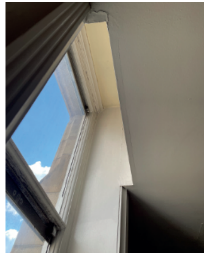
Inserted mezzanine floor window junction
