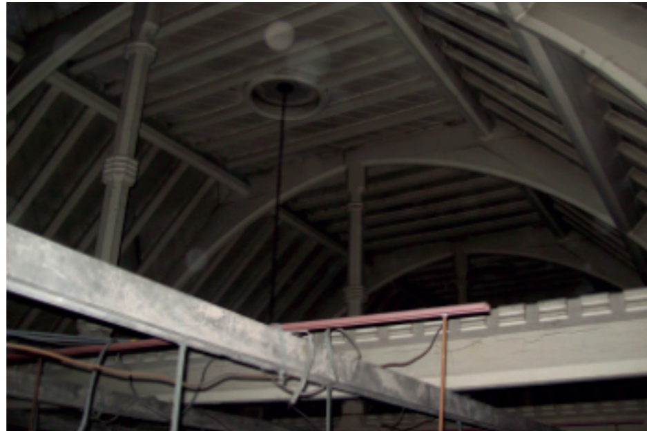
Eastern roof volume & original ceiling
