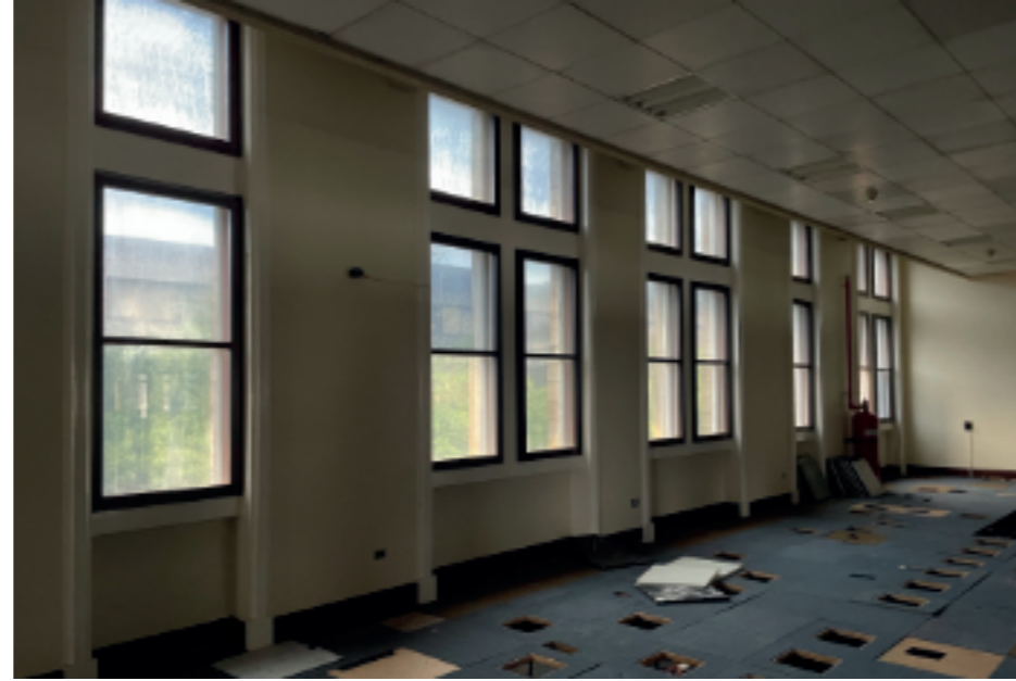
Computer Hall interior
