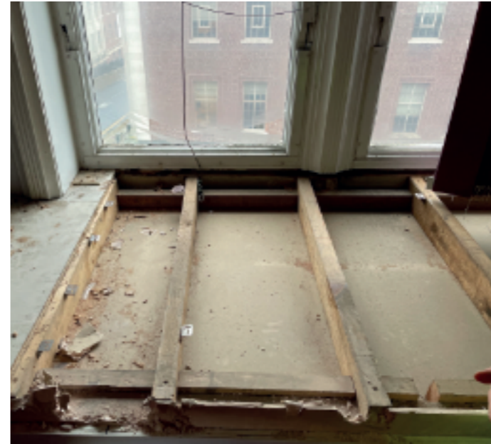
Opening up works to inserted floor step detail
