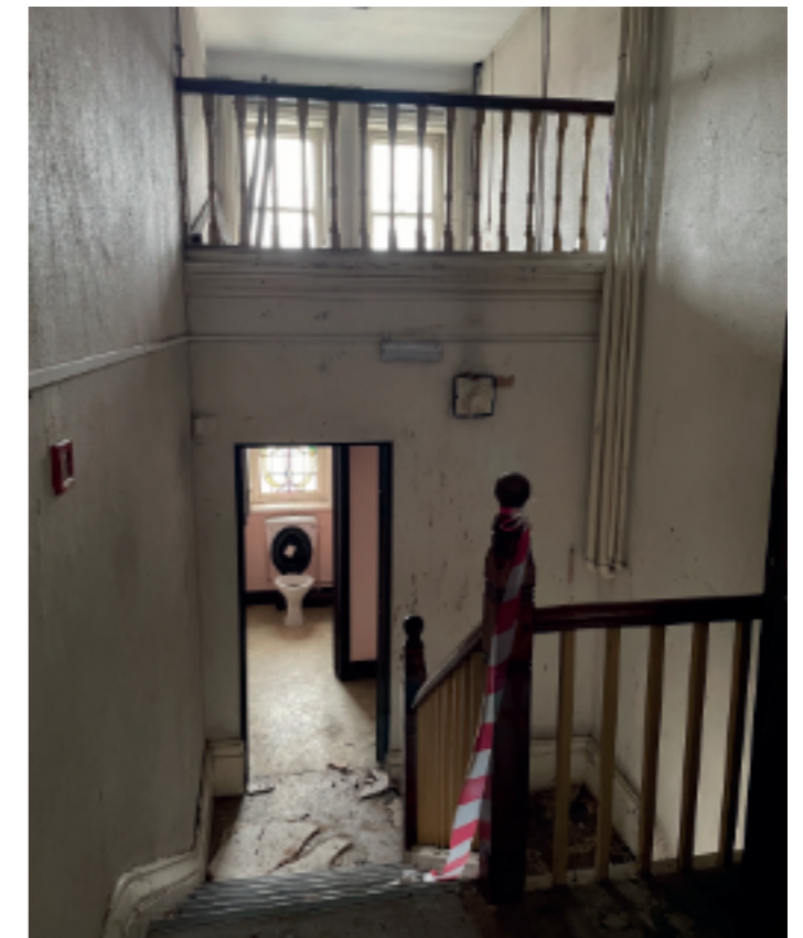
WCs to Northeast stair (below tower)
