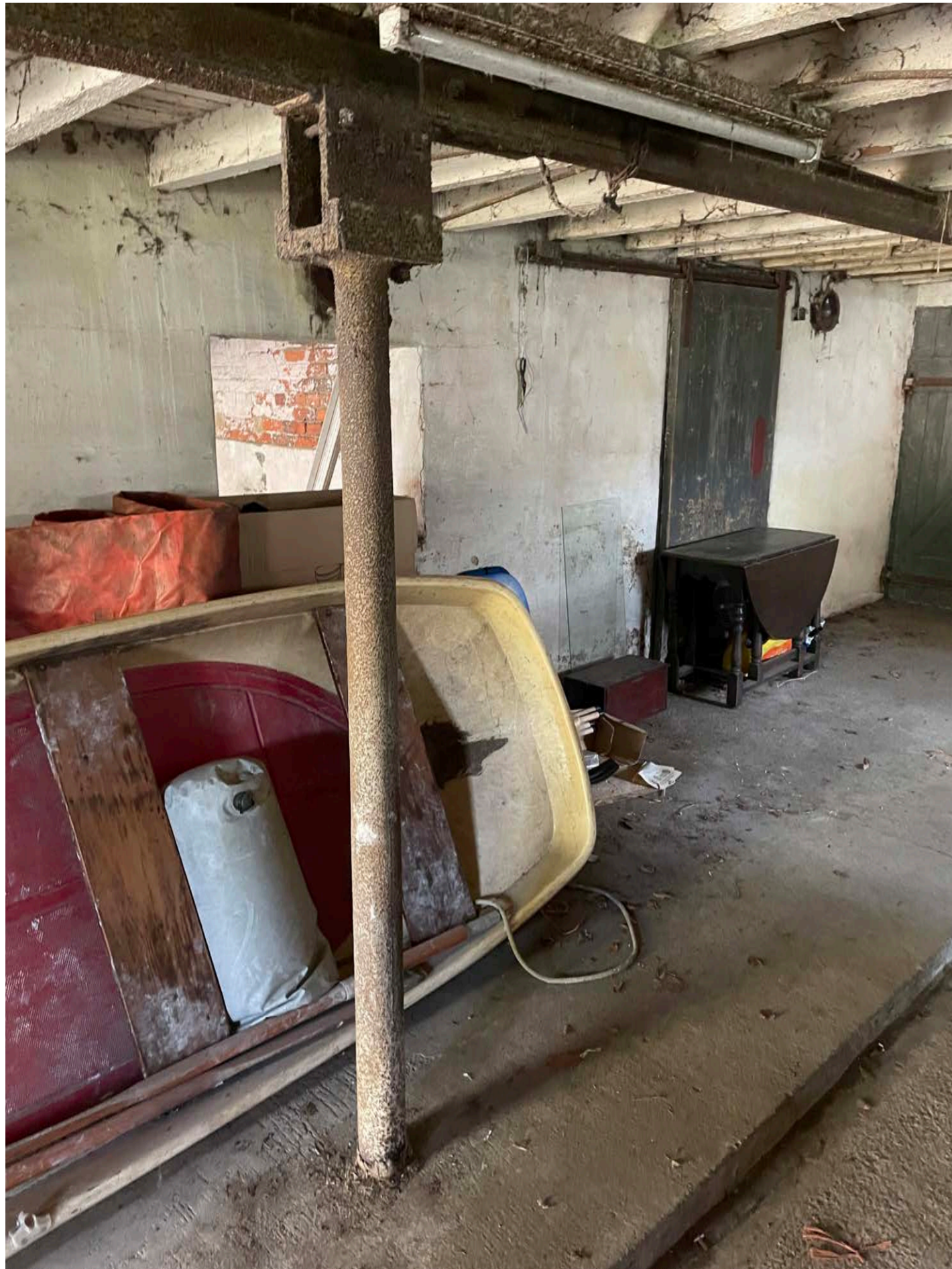
Photo Ref: E10 View of Nether Mill Barn (Internal Detailing First Floor Structure)
