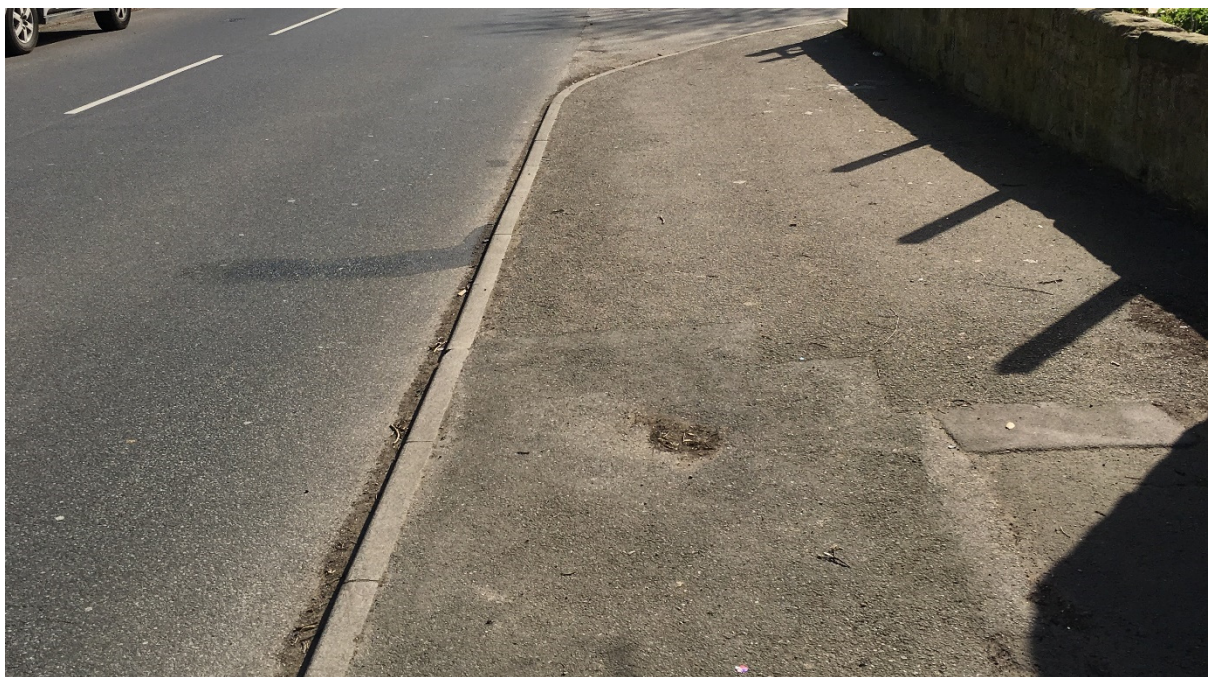
Figure 5 Eastern Side of Bell Mouth (Area 1)
