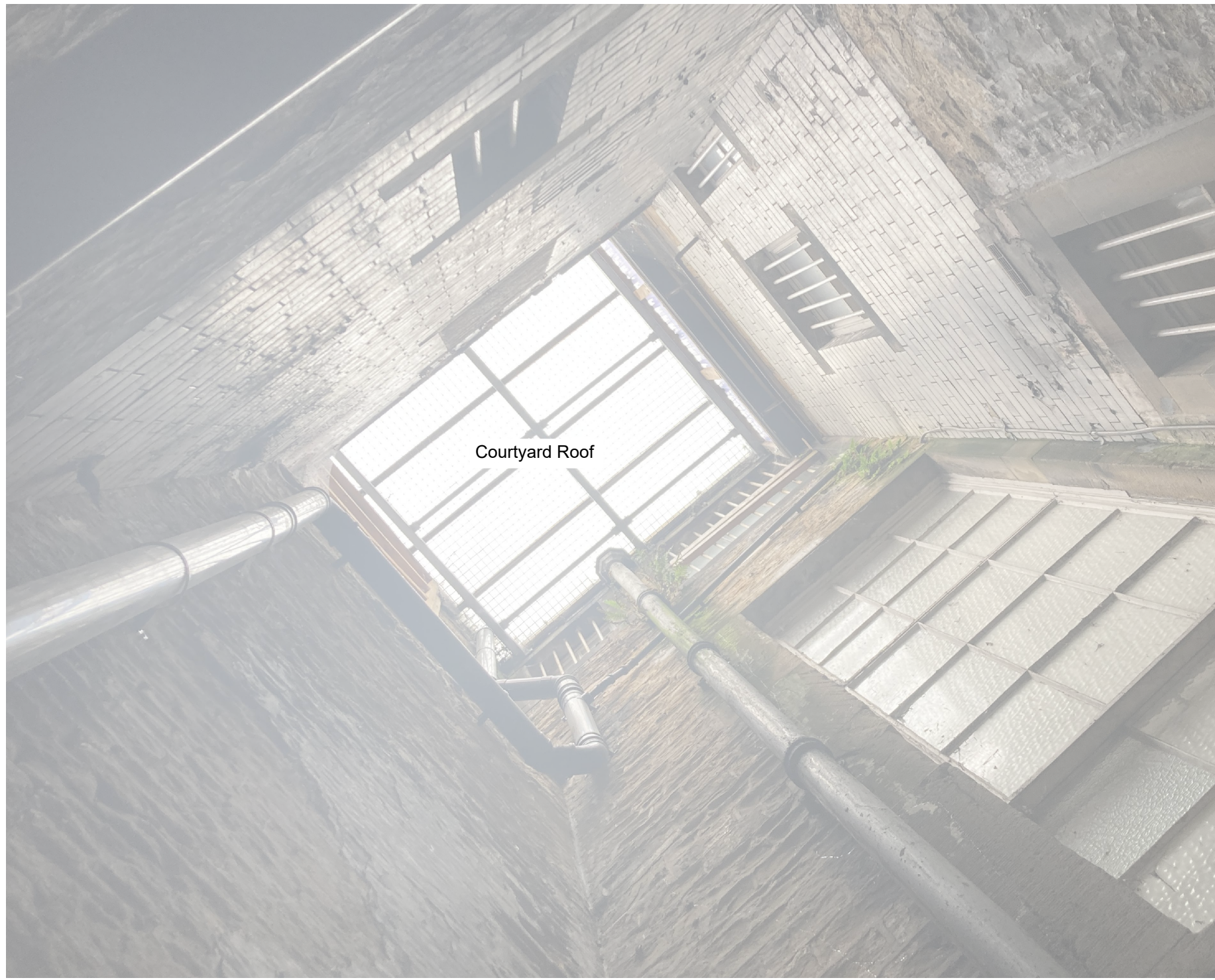
Courtyard Walls: Existing Not to scale
