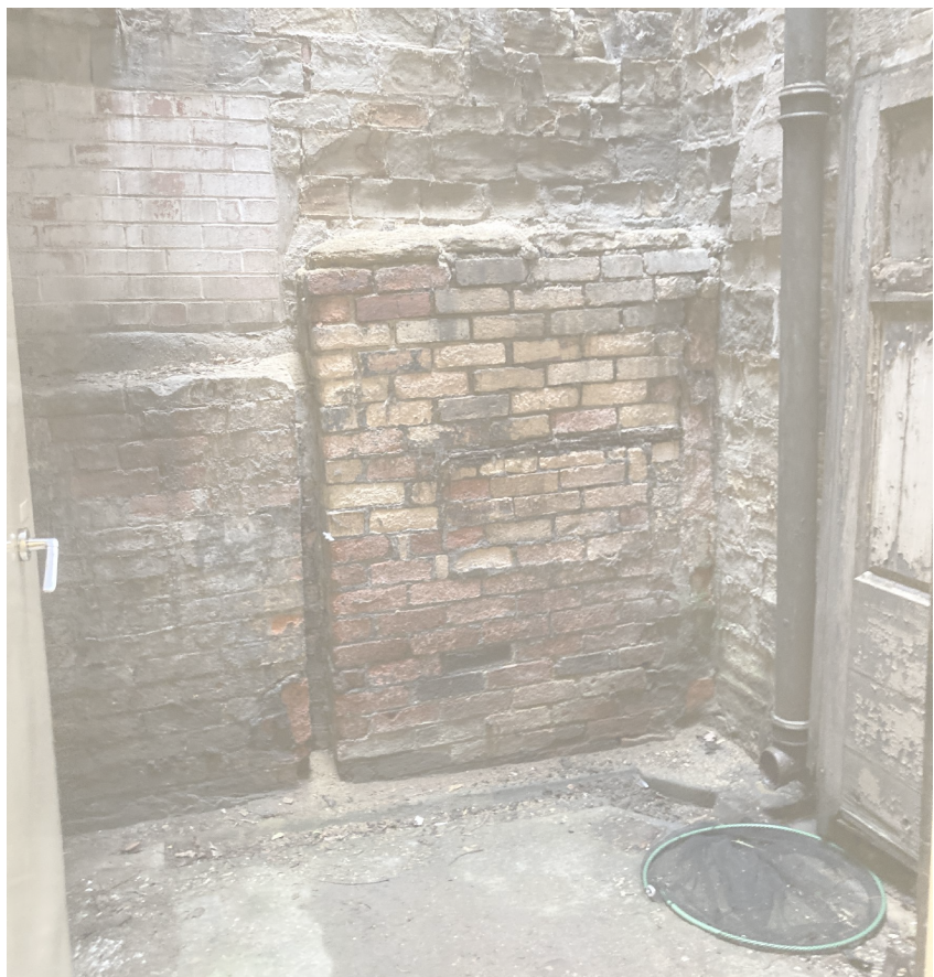
Courtyard Walls: Existing Not to scale
