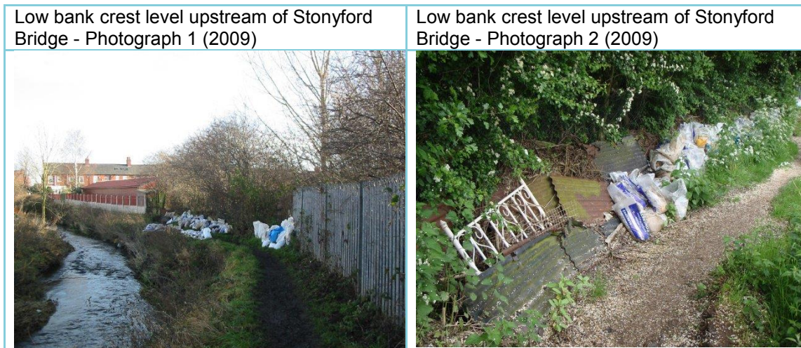
Figure 2-7: Stonyford Bridge photographs
