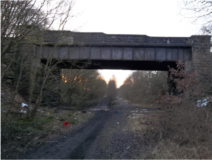
East elevation from track bed
