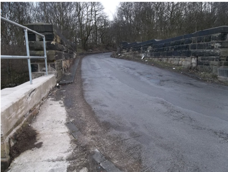
Existing Bridge deck looking south towards Darfield
