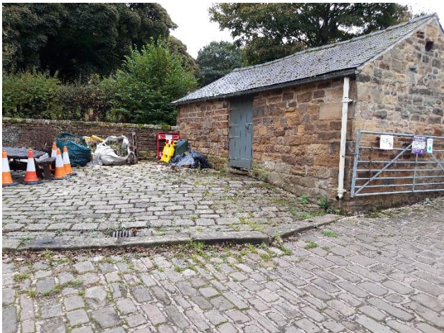
Existing levels within the Top Yard adjacent to outbuildings
