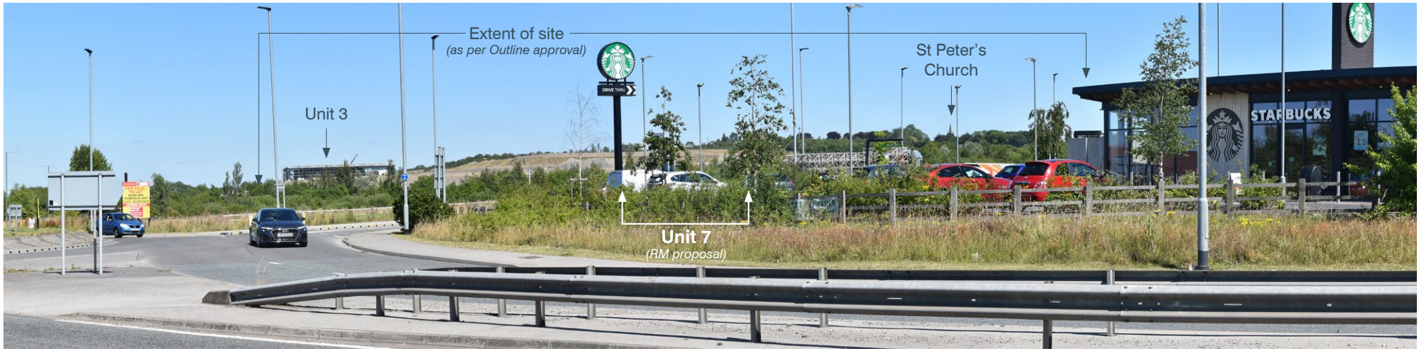
Viewpoint 21: Photograph taken on 22nd July 2024, showing the extent of the site, proposed Unit 7 location, local urban context and newly completed commercial development
