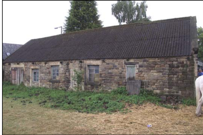
Plate 5: the north elevation of the Stable/Cartshed (building D) largely dates to the late 19 th century (prior to the fire)
