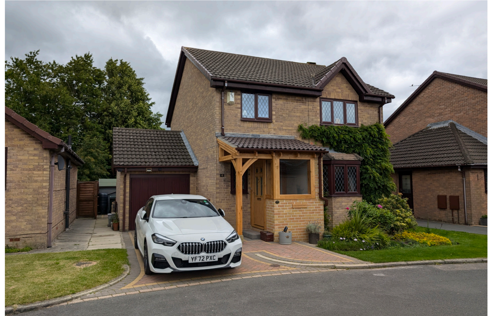
2403 - 4 Old Manor Drive, Oxspring, Sheffield, S36 8ZY Proposed (current) South-west (front) Elevation
