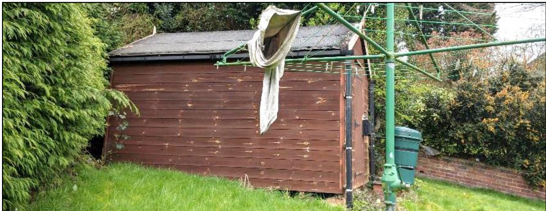
Plate 7. Southeast elevation of shed
