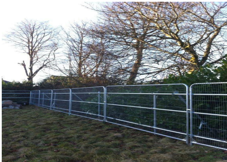
Photograph 1. Example of BS5837:2012 Protective Fencing
