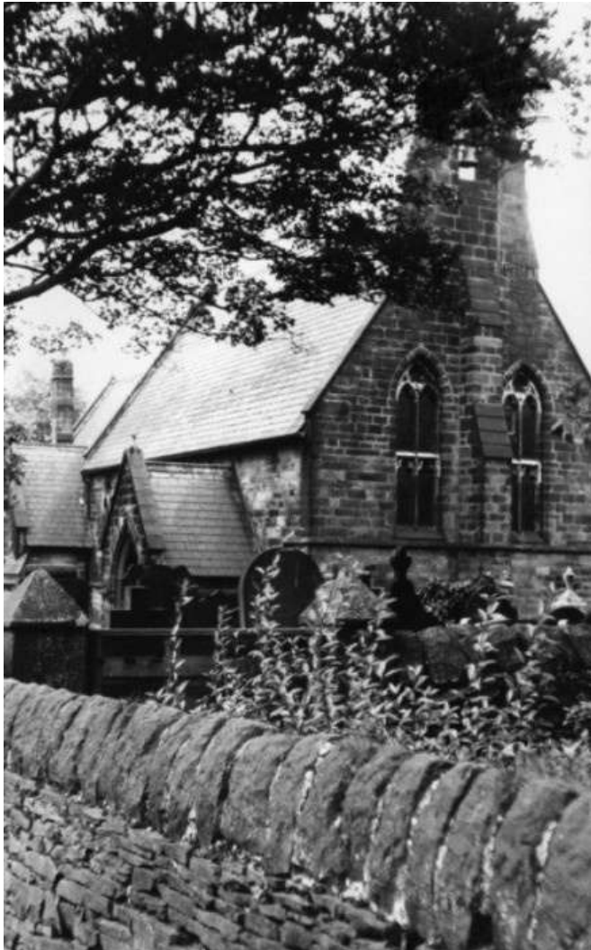
Fig 1. Holy Trinity Church (North-West Elevation) 1955. Source – Past Times in Thurgoland
