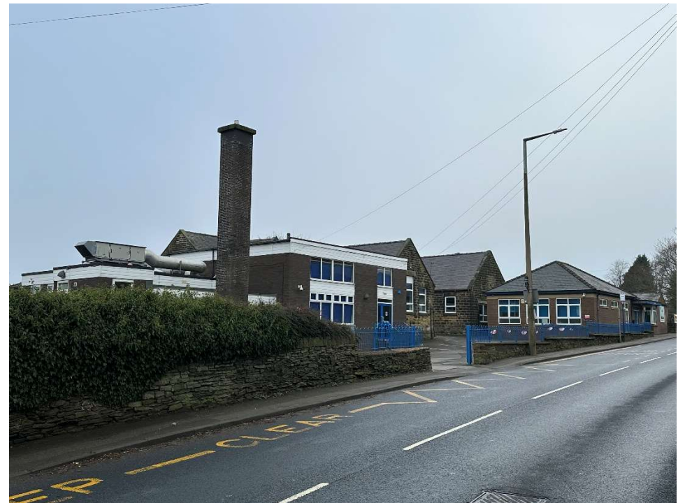
P13 – Looking from NE towards Thurgoland Primary School. Source: Photo taken on-site by author on 20.12.25.
