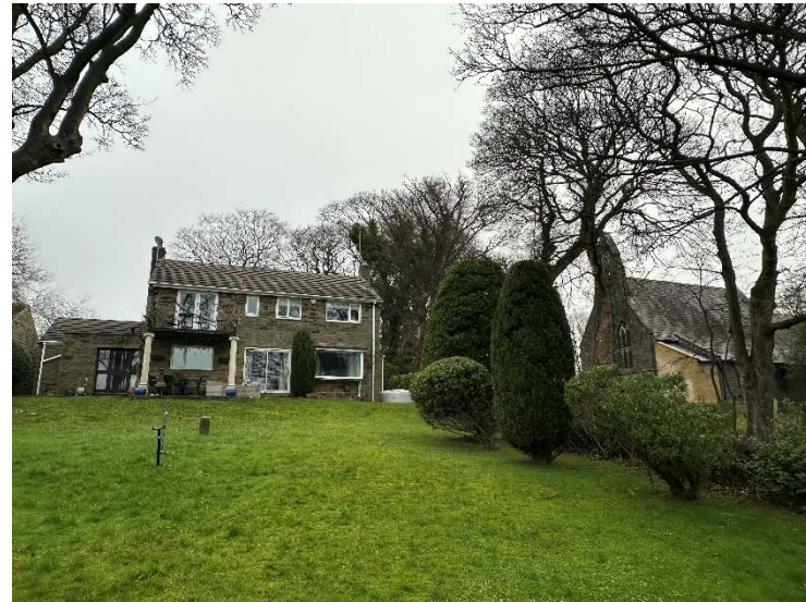
P11 – Looking from SW towards The Beeches and Holy Trinity. Source: Photo taken on-site by author on 20.12.25.
