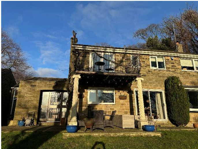
P16 – Existing South Elevation to The Beeches identifying first-floor balcony and columns to be removed. Photograph by D. Houlty, Dec 2025.
