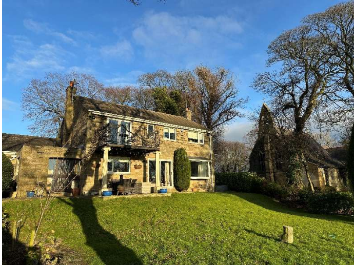
P14 – Existing south elevation to The Beeches and Holy Trinity Church Photograph by D. Houlty, Dec 2025.
