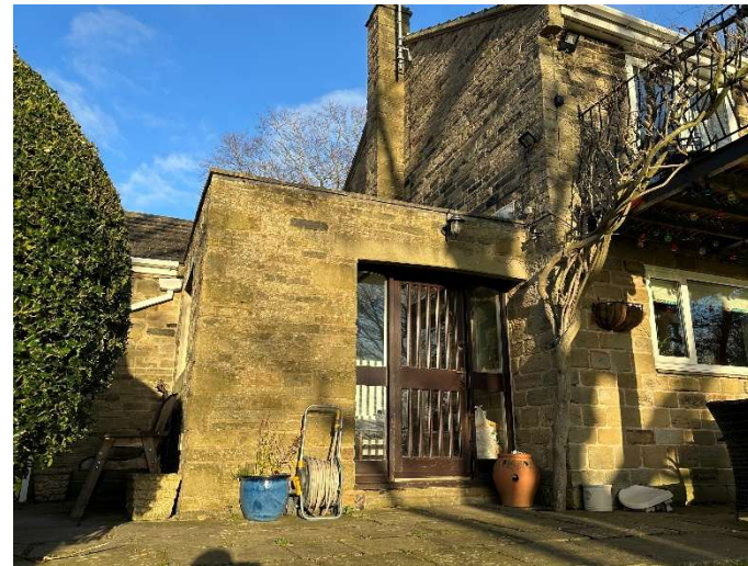
P17 – Existing South Elevation to The Beeches identifying 1980's 2.5x2.5m extension to be removed. Photograph by D. Houlty, Dec 2022.
