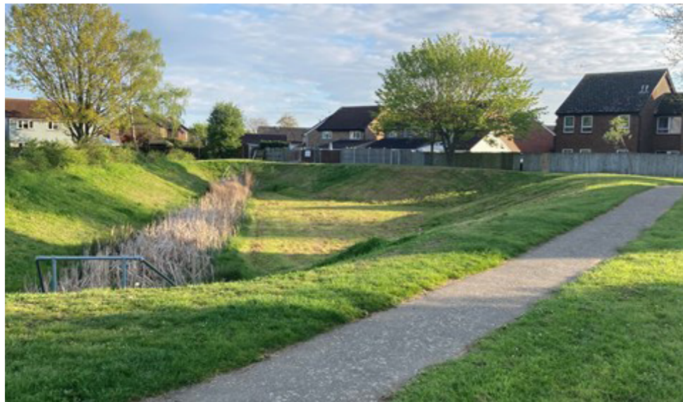
Example of dry detention basin
