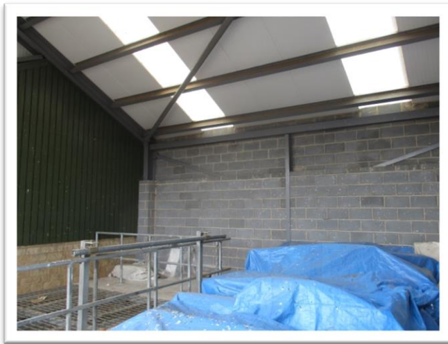
Internal of the hopper building
