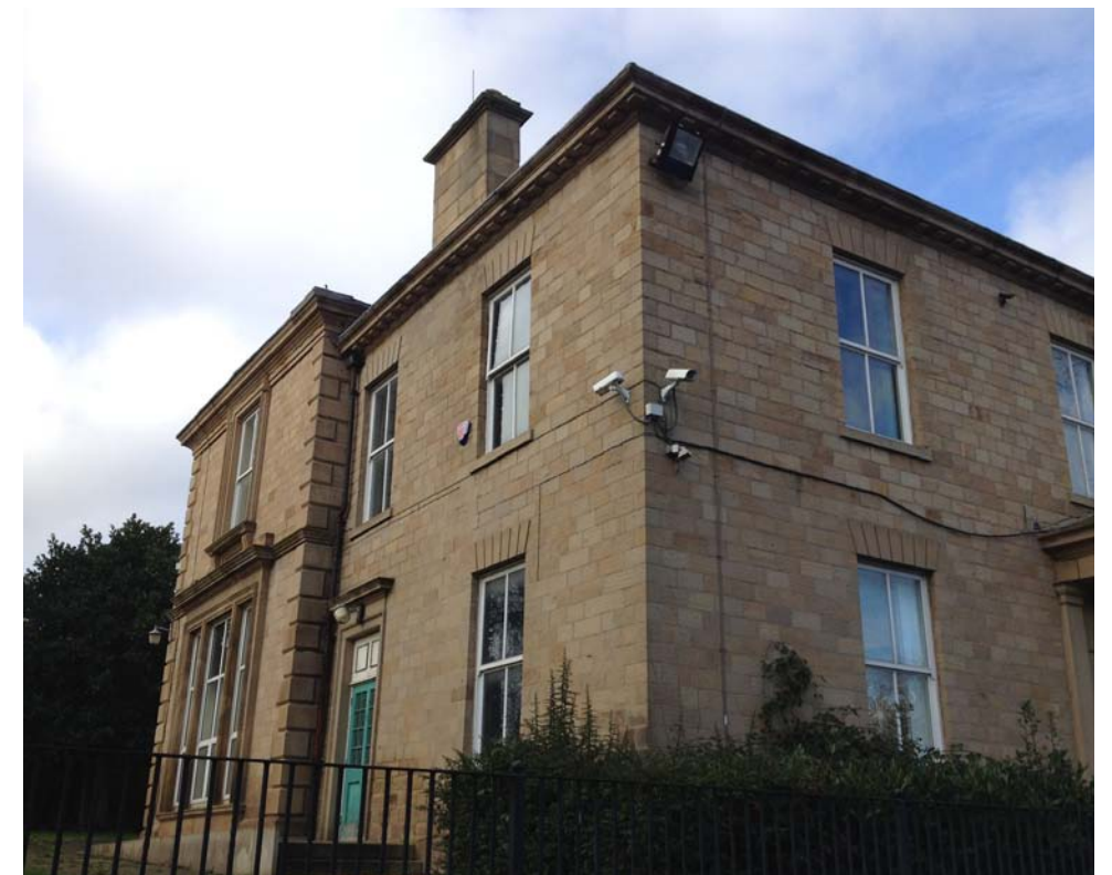
Image 9; Belle Vue House displays dressed stone and coining details.
