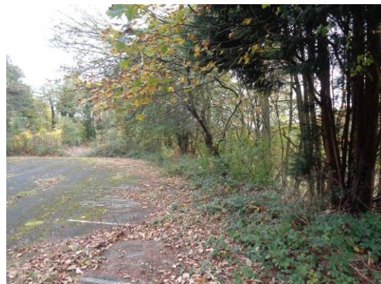
Plate 4: Upper car park showing proximity of poor grade trees to hard standing requiring removal
