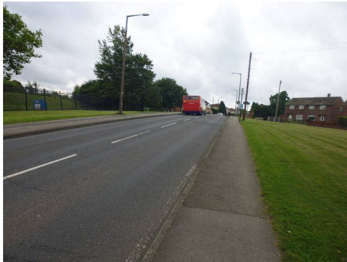
Photo 7: Pedestrian Infrastructure on Carlton Road
