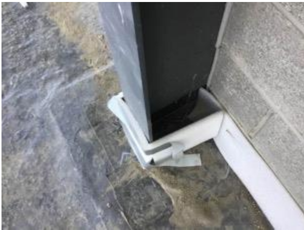
Sealed stanchion detail
