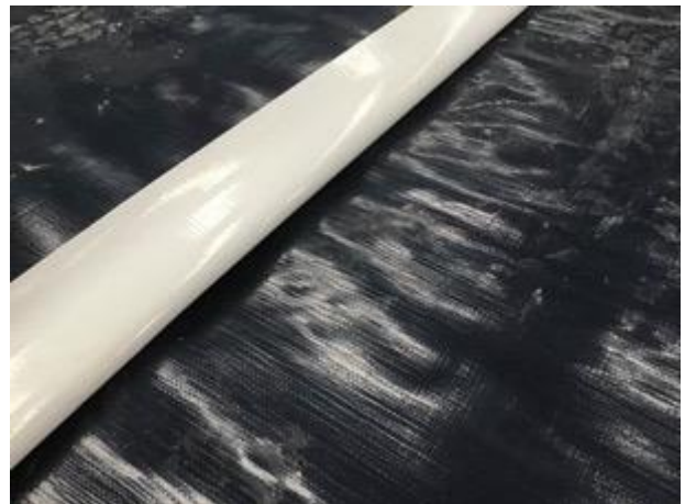
Sealed membrane tape joint
