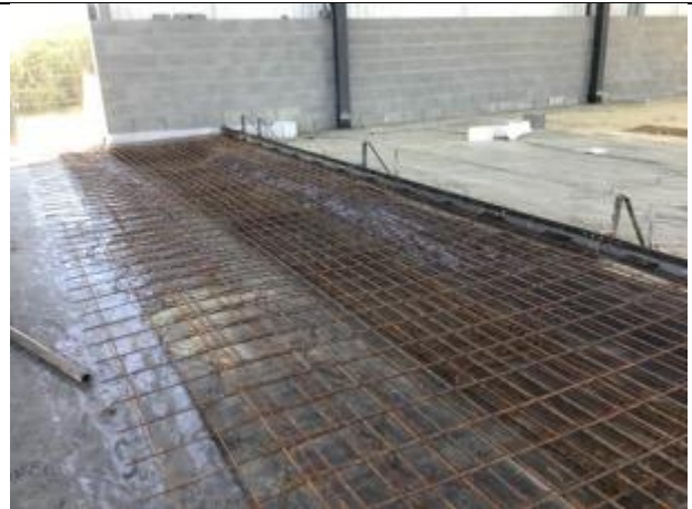
Thickening area restricted inspection
