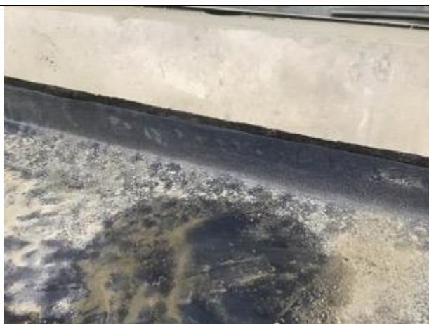
Sealed perimeter detailing
