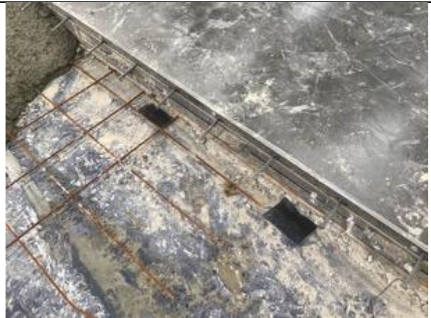
Sealed SAGM patch repairs
