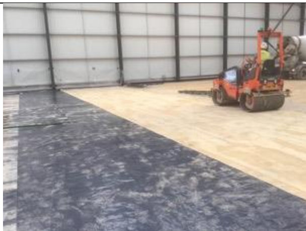
Ground being rolled, membrane laid
