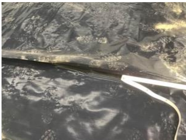
Joint using double sided joint tape
