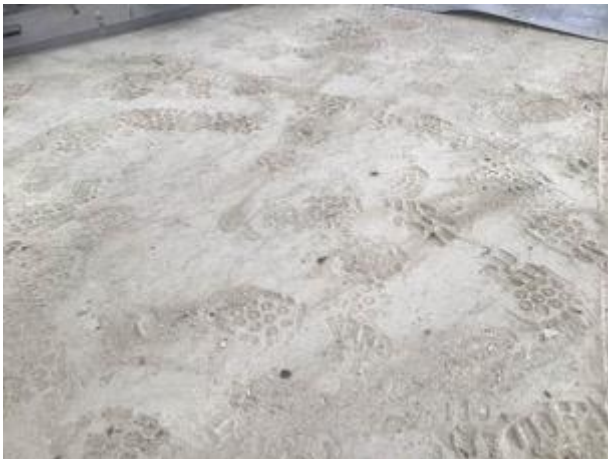
Sand blinding sub grade prior to being rolled
