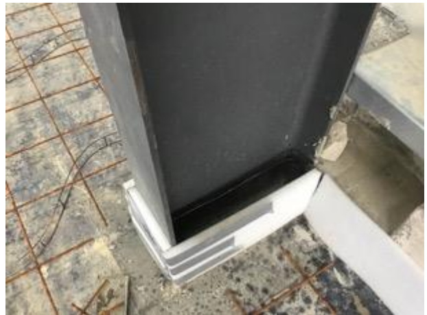
Sealed stanchion detail
