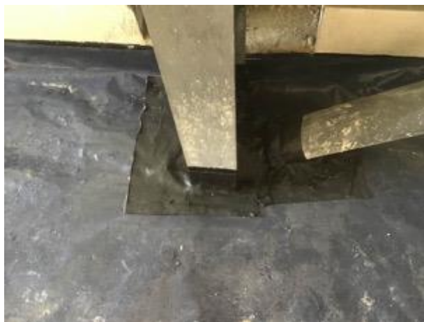
Stanchion seal using SAGM
