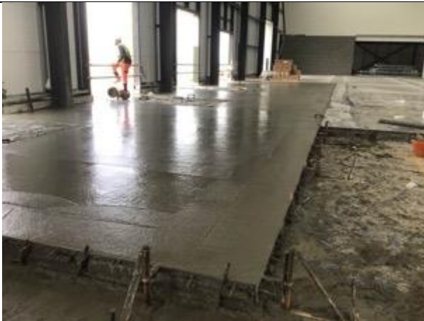
Dock levellers poured prior to our arrival
