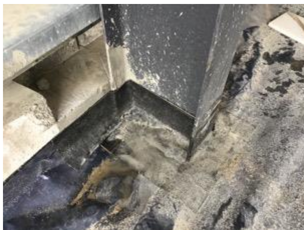
Sealed stanchion detail
