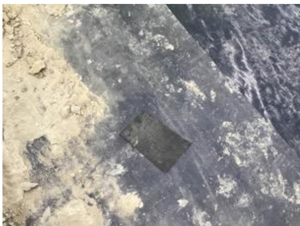
Sealed SAGM patch repair
