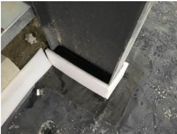
Sealed stanchion detail with miothene installed by others
