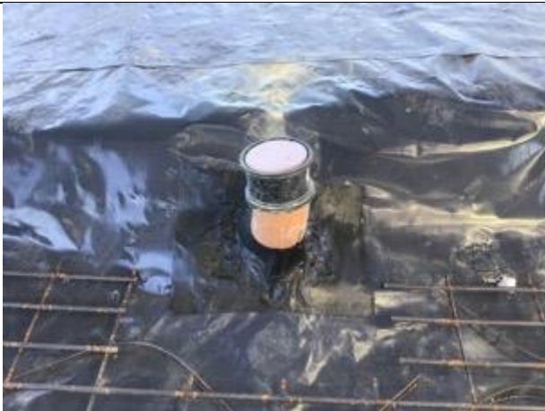
Sealed pipe penetration
