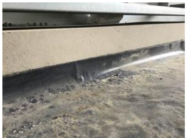
Sealed perimeter detailing
