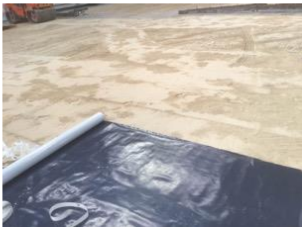
Membrane being rolled out
