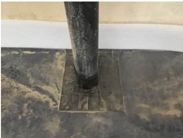
Sealed pipe penetration
