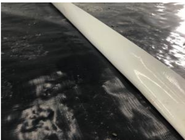
Sealed double sided tape joint
