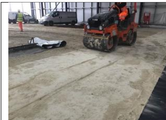
Sub grade prep
