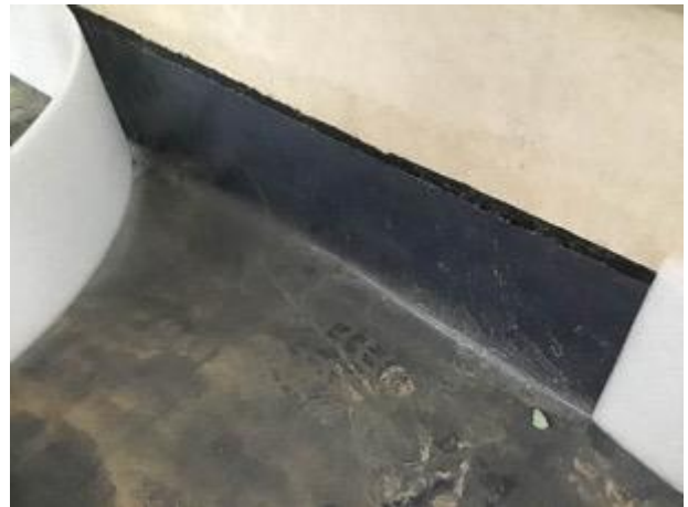
Sealed perimeter detailing
