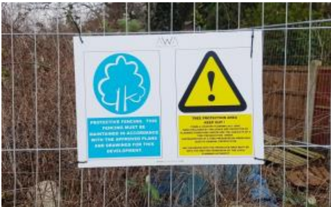
Example of A3 Correx tree protection warning sign fixed to fencing panel
