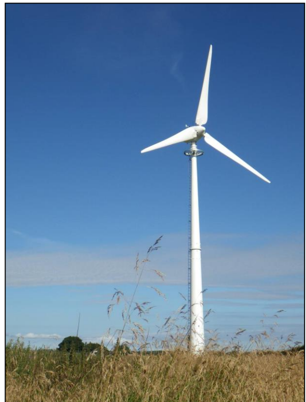
Photograph showing existing Earthmill turbine on open arable land
