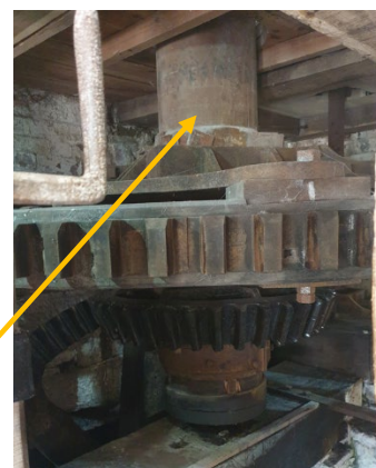
Lower part of upright shaft
