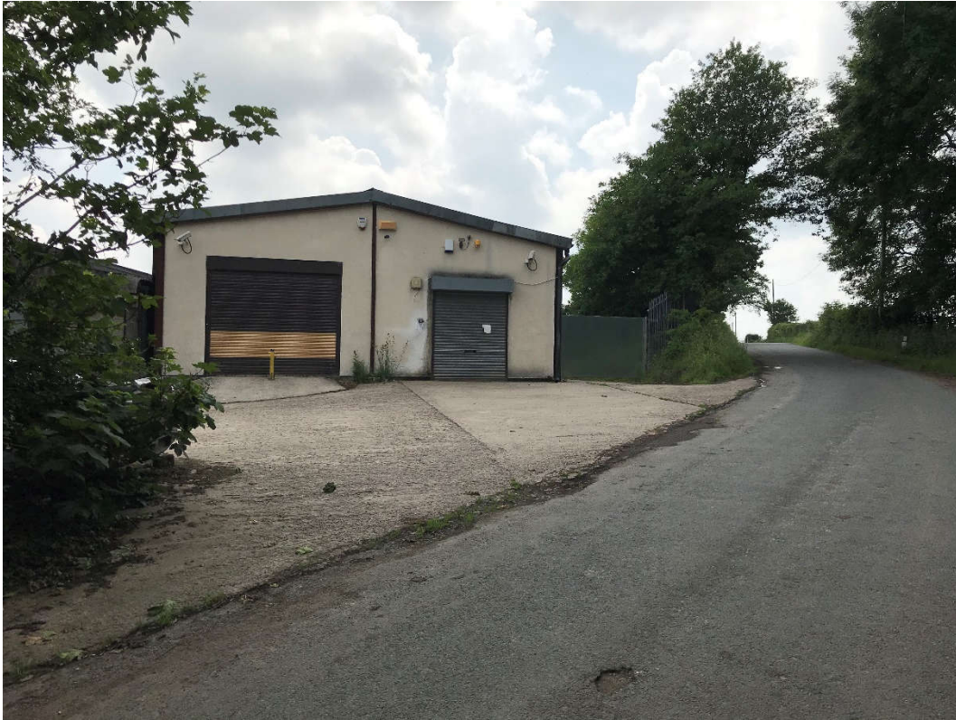
Fig 11. Existing access to Stainborough Lane.
