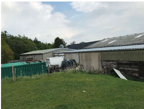
Fig 05. View of Building A from S West
