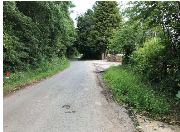
Fig 13. View from access looking n-east.
